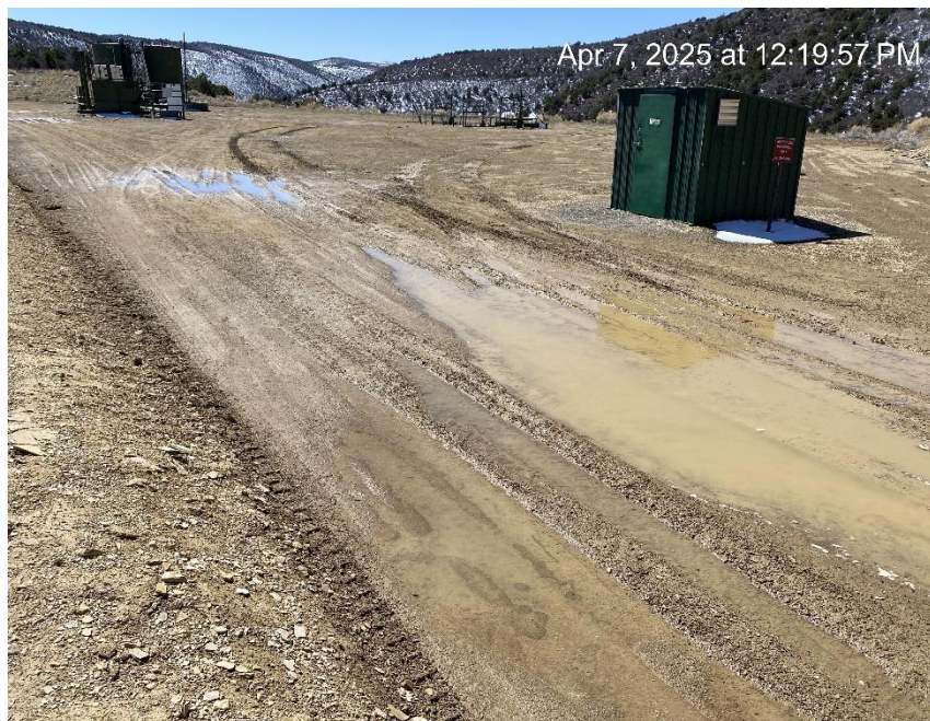
Location from North entrance
