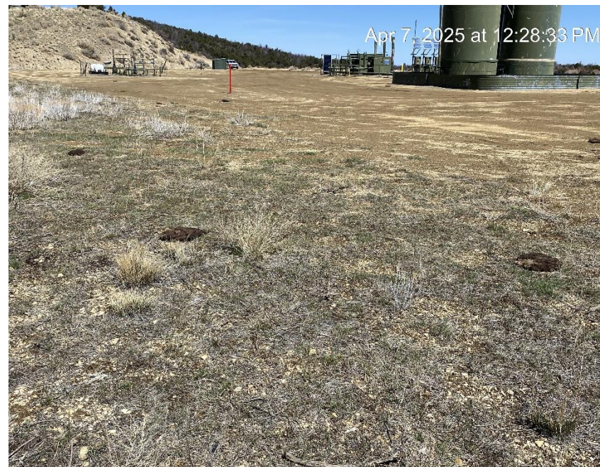
Location from South corner
