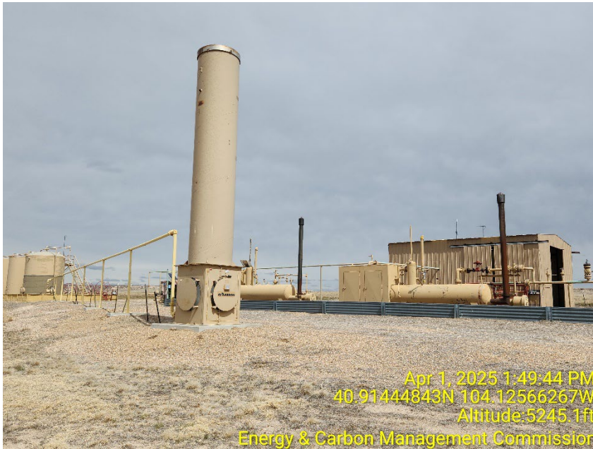
Photo 3 – ECD and Separators
