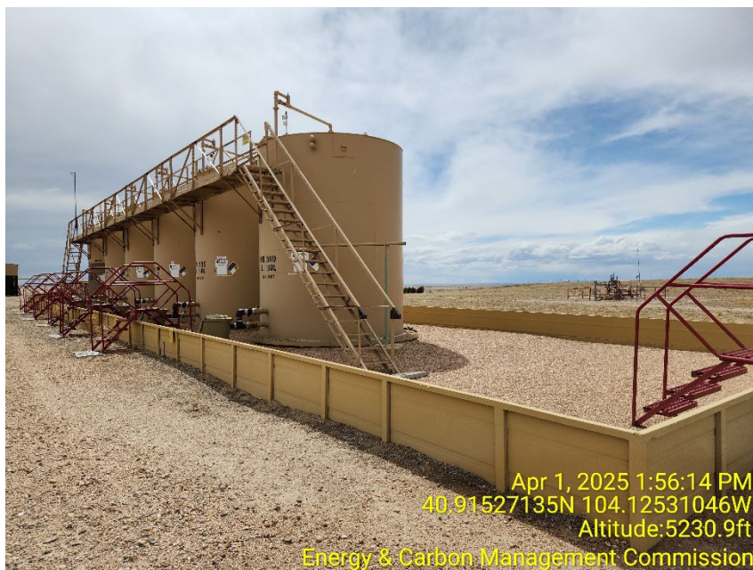
Photo 9 – Tank Battery – Sign missing
