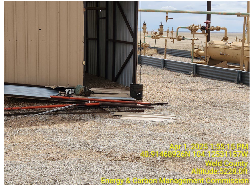
Photo 6 – Unused parts at Compressor Building
