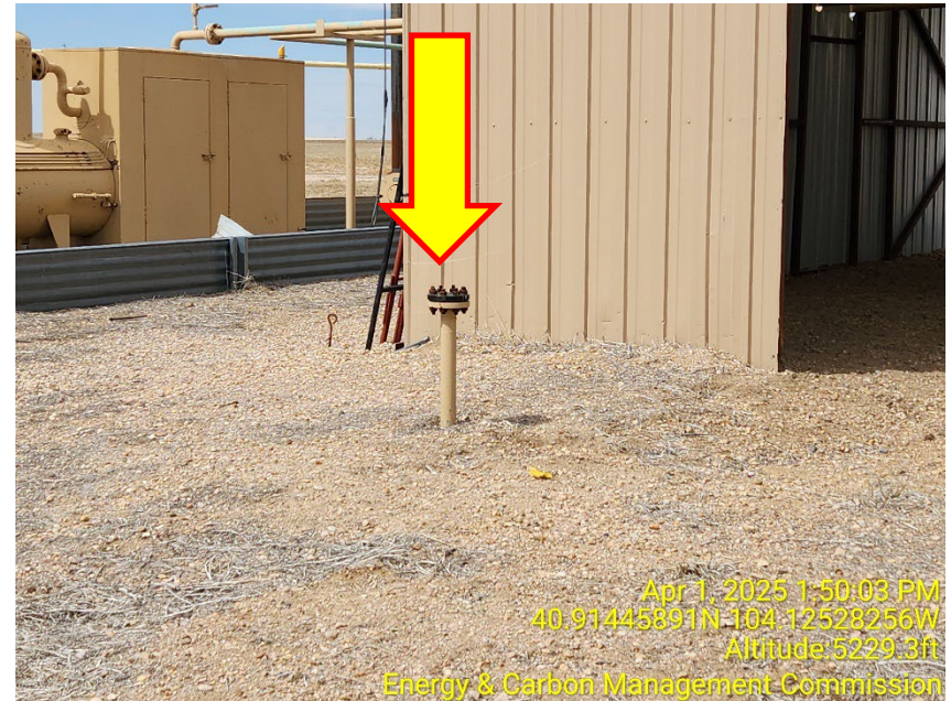
Photo 4 – Unmarked Riser
