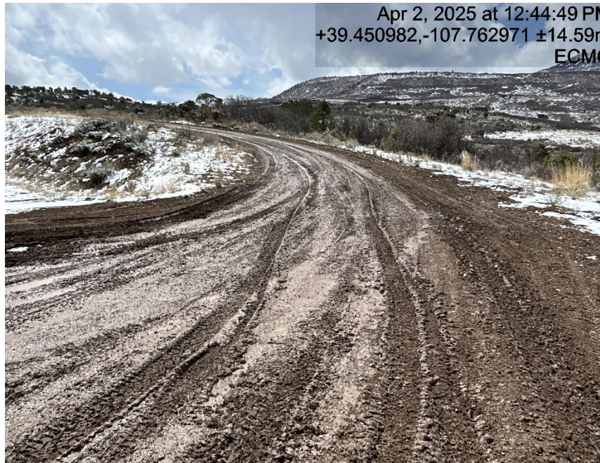
Lack of stabilization/compaction and no tracking BMP's observed.
