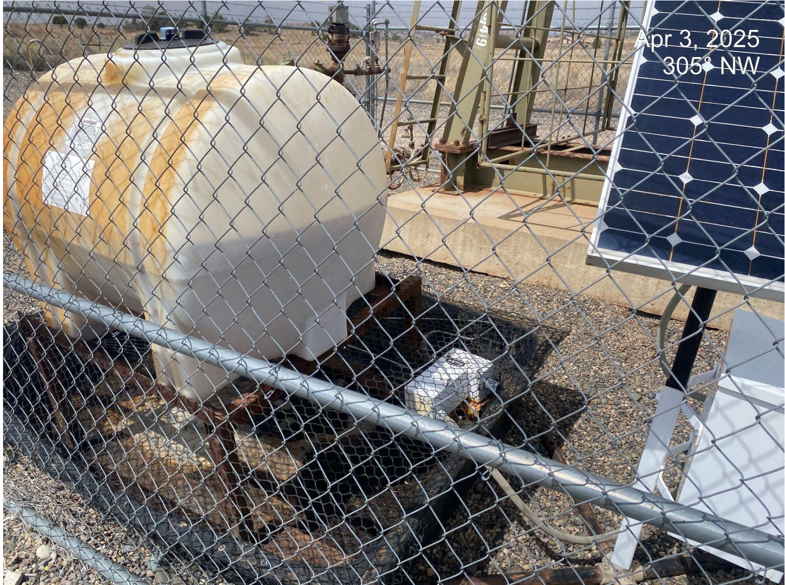
Photo 2. Wildlife netting has been installed at chemical tank secondary containment.
