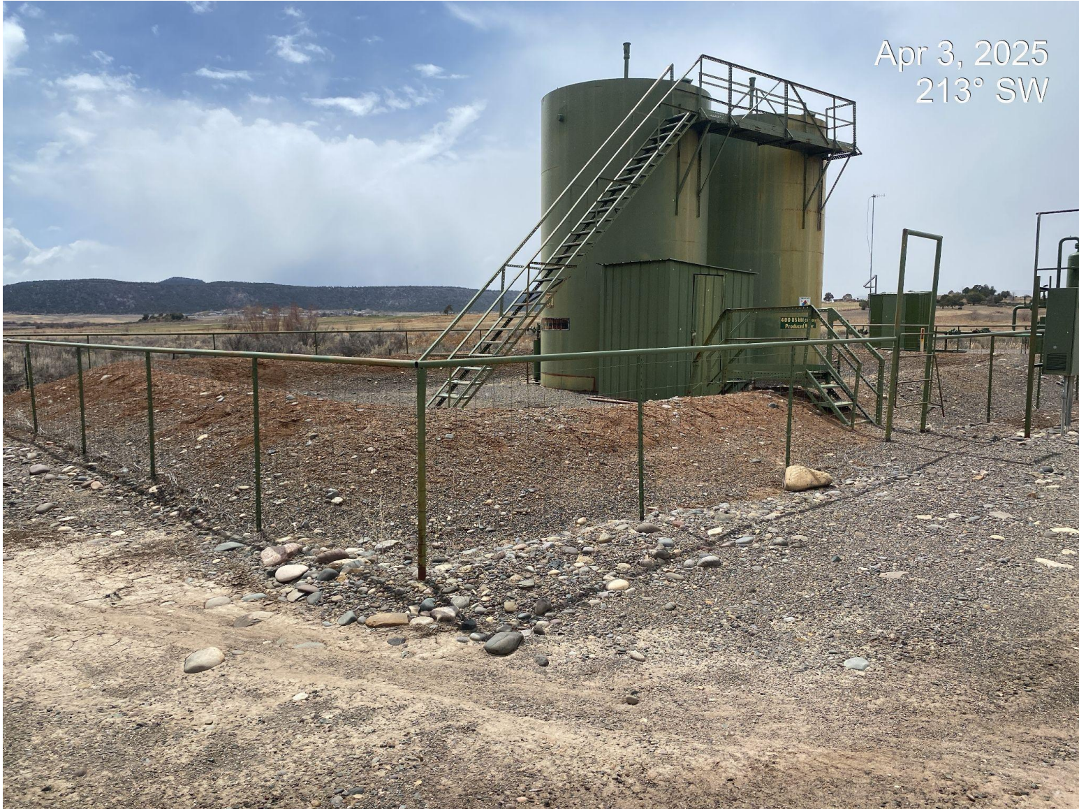
Photo 4. Weedy debris have been removed from produced water tank berms.
