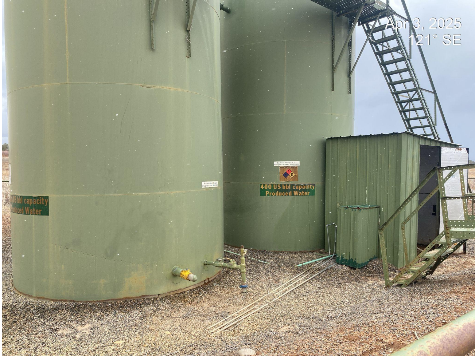
Photo 3. Current operator not displayed on produced water tanks. "Southland Royalty" still displayed.
