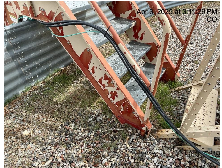
Photo # 9059 Weeds in secondary containment
