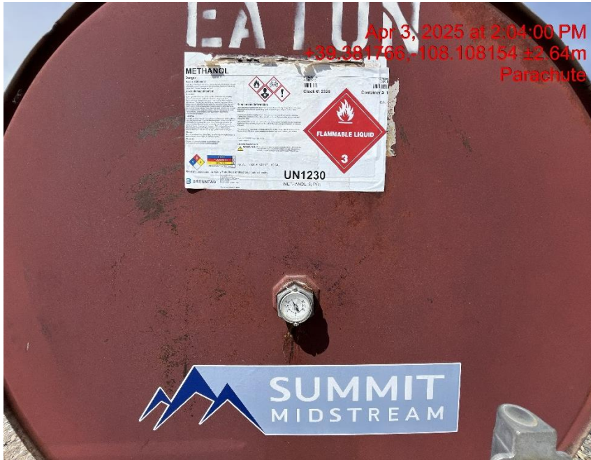
Photo # 6936 Methanol tank lacks required labeling/does not comply with CECMC rules
