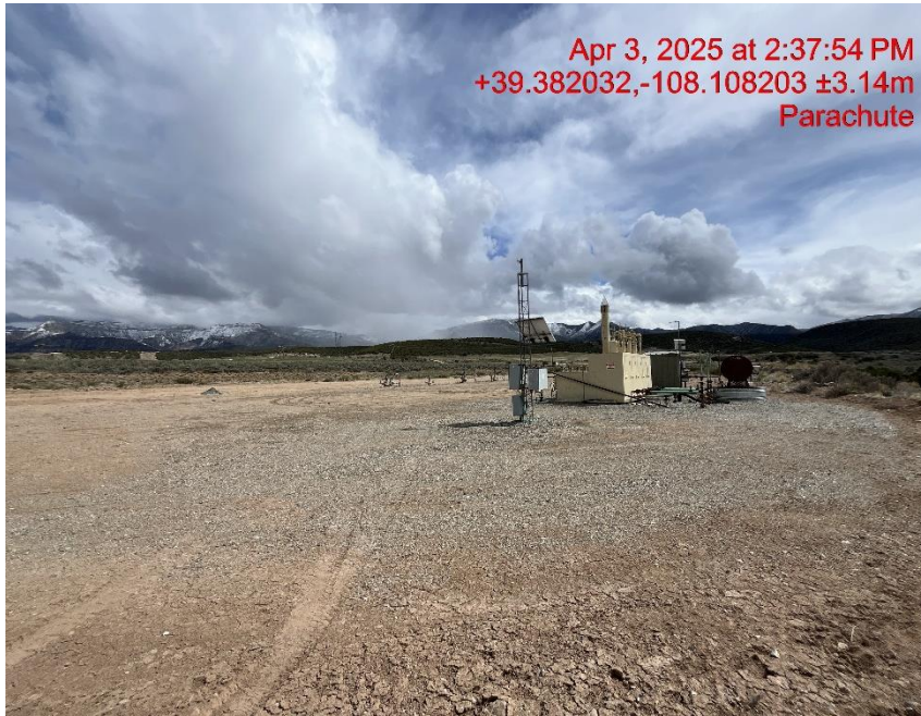
Photo # 6954 NW corner of location
