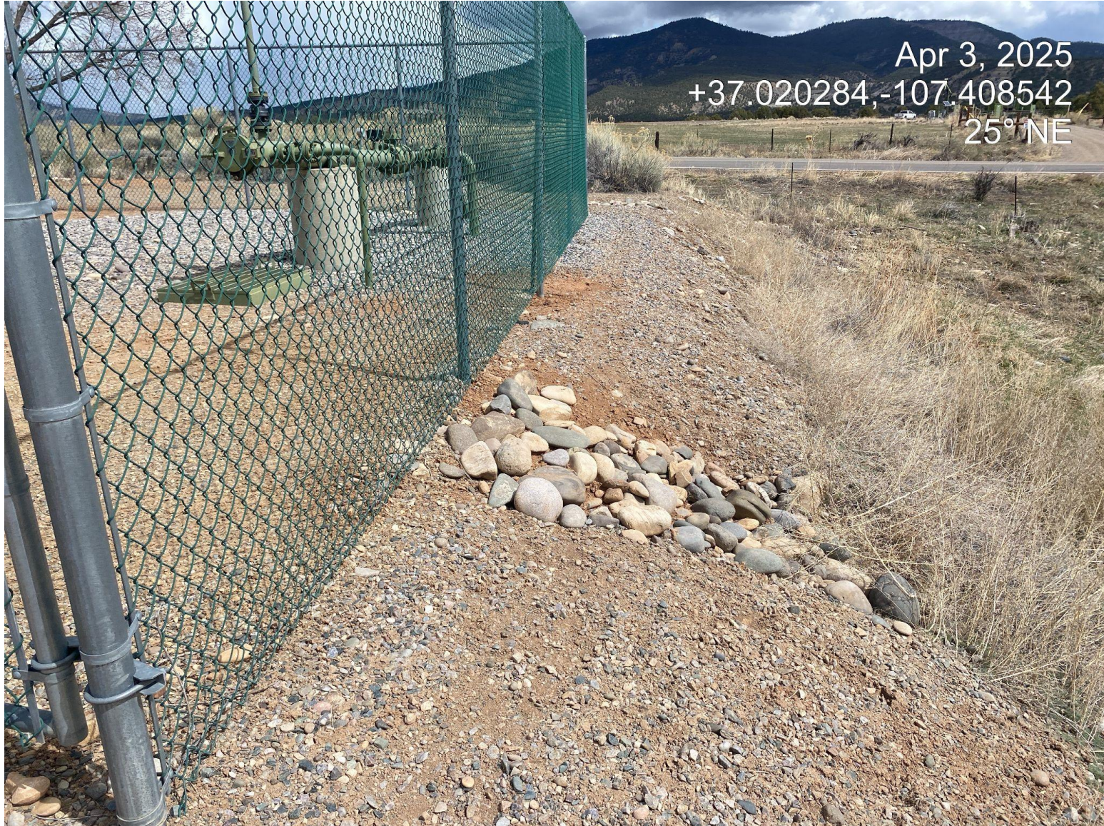
Photo 4. Stormwater BMPs installed in the eastern portion of the location.
