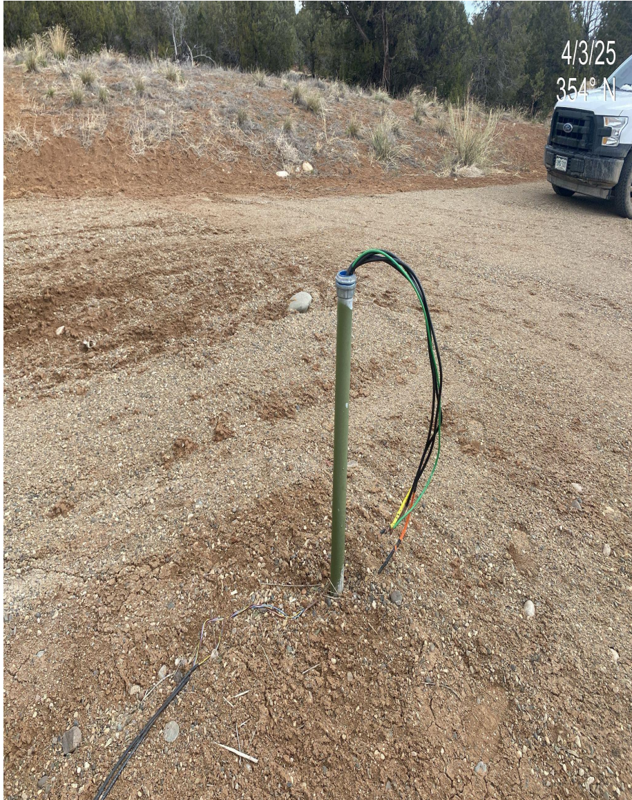
Photo 4. Disconnected, unused exposed wires observed on the northern edge of the pad.
