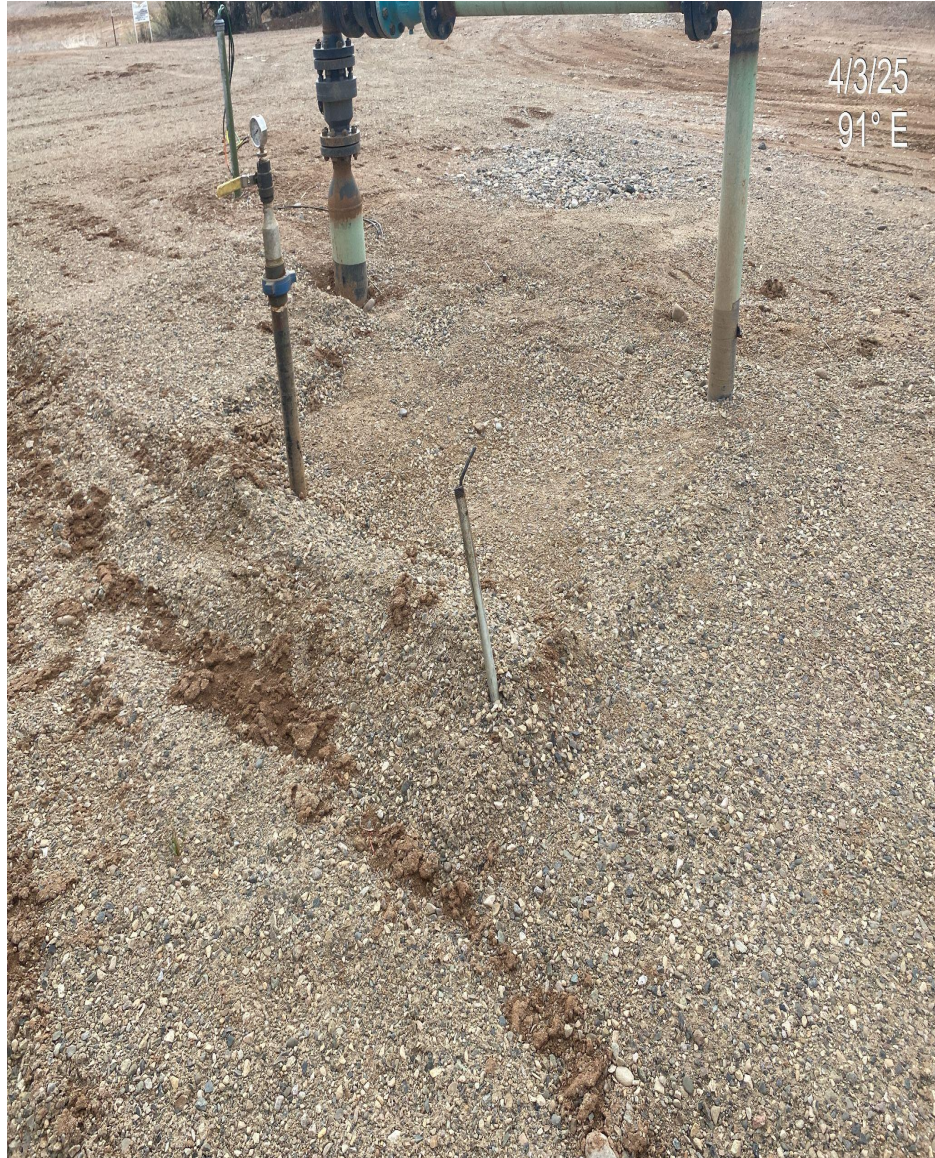
Photo 4. Disconnected, unused exposed wires observed on the northern edge of the pad.
