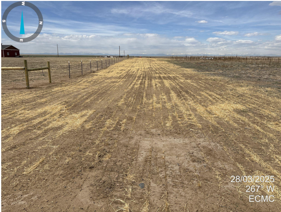
Photo 1. Looking west down access road. It appears that reclamation has been conducted with evidence of crimped straw.
