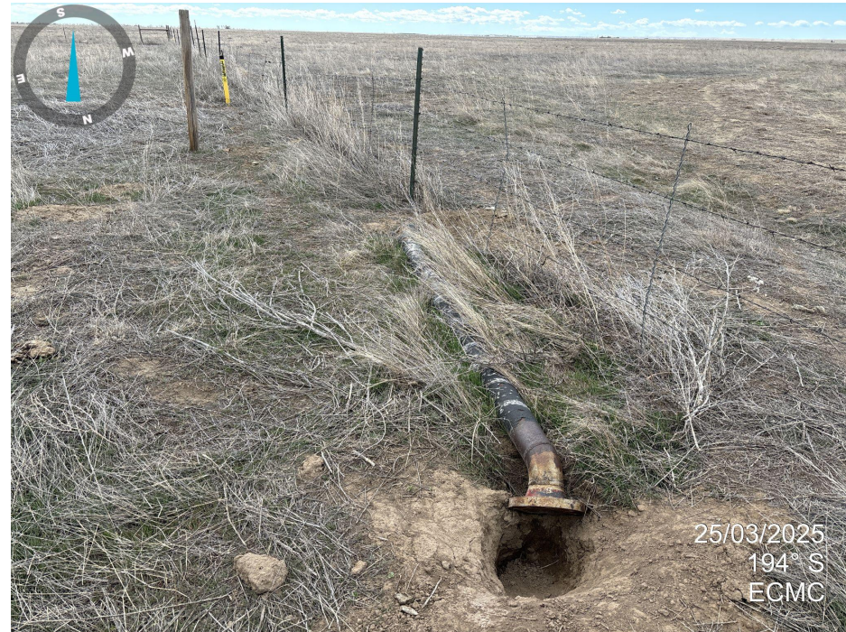
Photo 6. Picture taken on the west side of location, middle. Pipe remains on location.
