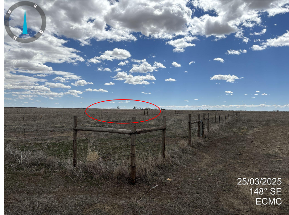
Photo 6. Picture taken at the northwest corner of location. Location is fenced. A large wire gate was down at time of inspection (red circle).
