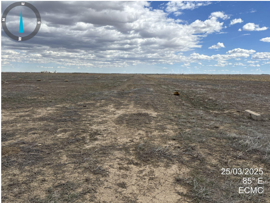
Photo 1. Looking east down access road from well API 001-07450. Vegetation coverage on road is lower than surrounding area and primarily undesirable weedy vegetation.
