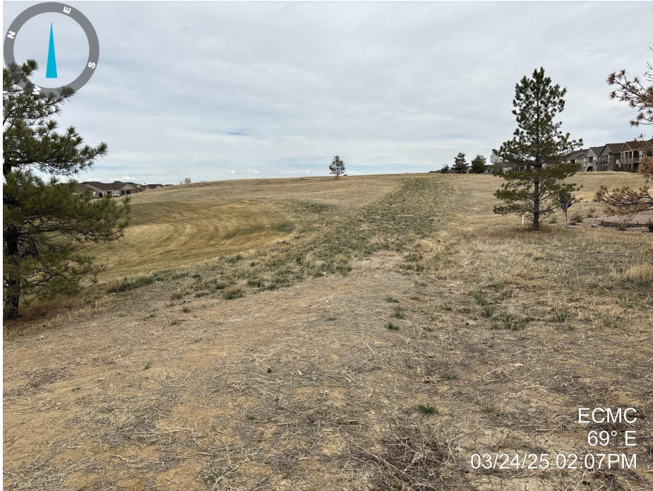
Photo 5. Photo taken from the start of the access road, facing East. Photo illustrates that the access road has been reclaimed, but at the entrance to the access road, bare soil patches remain.
