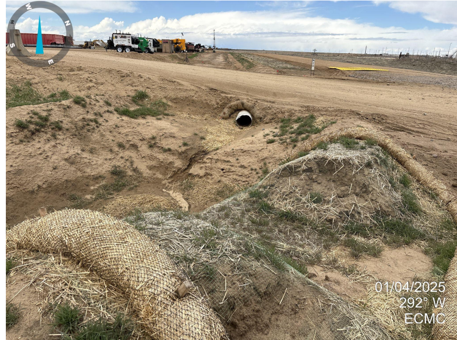
Photo 4. Picture taken at northeast corner sediment trap. Outflow BMP are in place. A small amount of erosion is beginning to form under the culvert.
