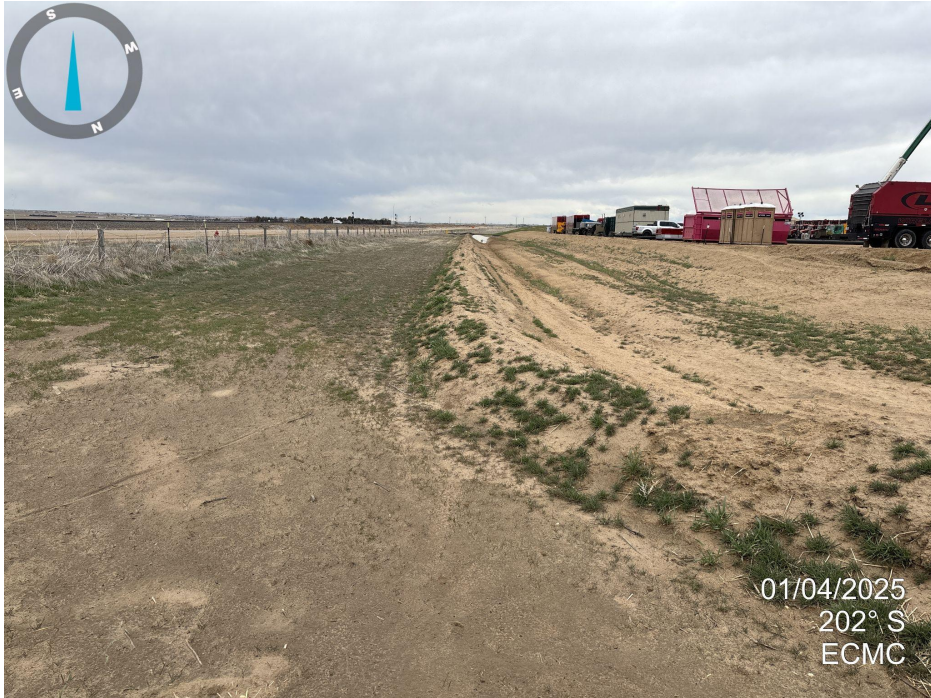
Photo 5. Looking south down the east side of location. Ditch appears stabilized.
