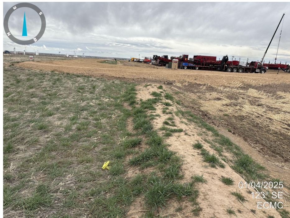
Photo 16. Looking east down north side of location. Ditch is present and appears to be stabilized.
