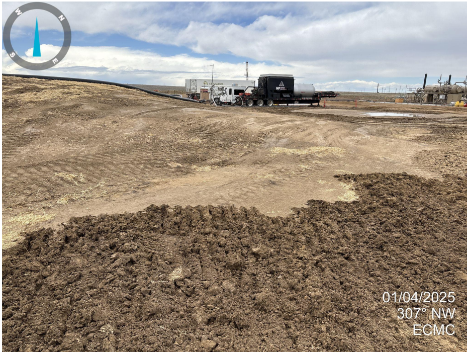
Photo 11. Looking at the northwest corner of the triangular topsoil stockpile towards the production facility. It appears that equipment has been driving over the corner of the topsoil stockpile.
