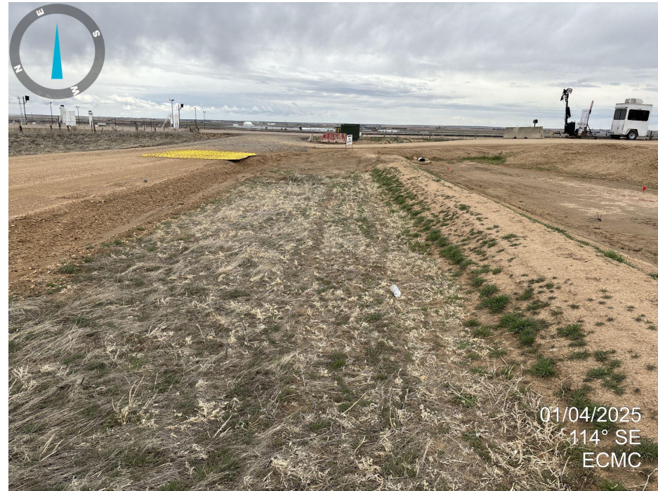
Photo 2. Looking east down access road. A track out mat is present on the outboard lane. Culvert under access road has inlet protection.
