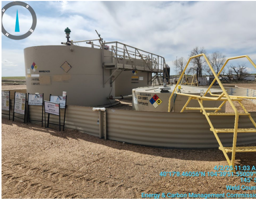
Photo 3: Centralized tank battery
