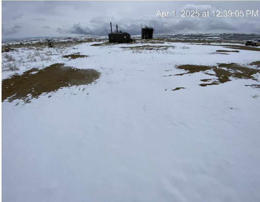
Location from North corner
