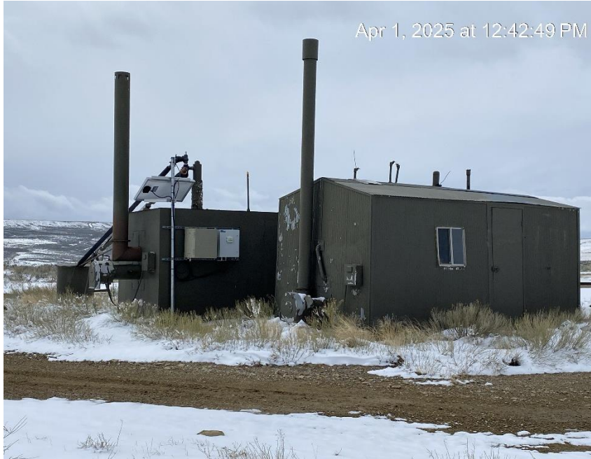
Unused equipment in foreground
