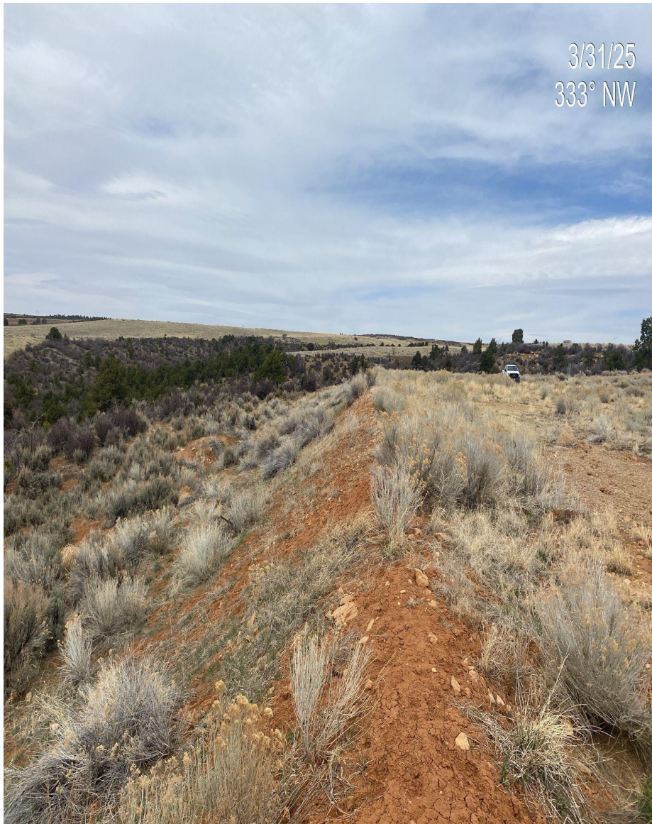
Photo 2. View of location fill slopes. Slopes have establishment of desirable vegetation including but not limited to Crested Wheatgrass, Sand Dropseed and Rabbitbrush.
