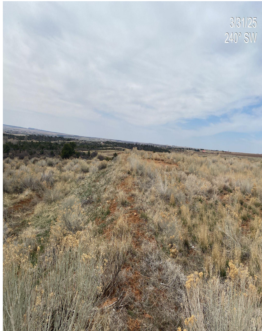
Photo 2. View of location fill slopes. Slopes have establishment of desirable vegetation including but not limited to Crested Wheatgrass, Sand Dropseed and Rabbitbrush.
