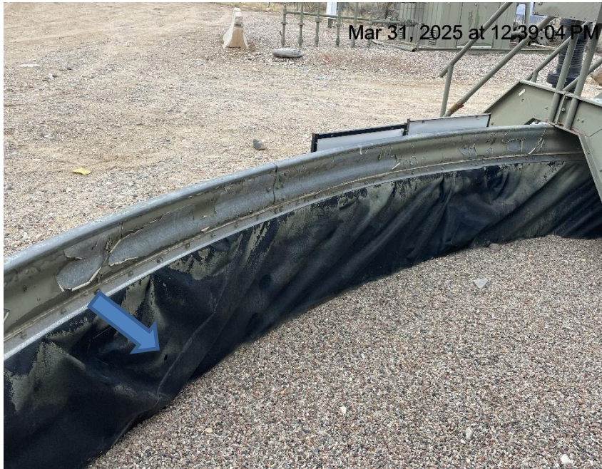
Photo # 8402 Hole in secondary containment liner/liner needs maintenance
