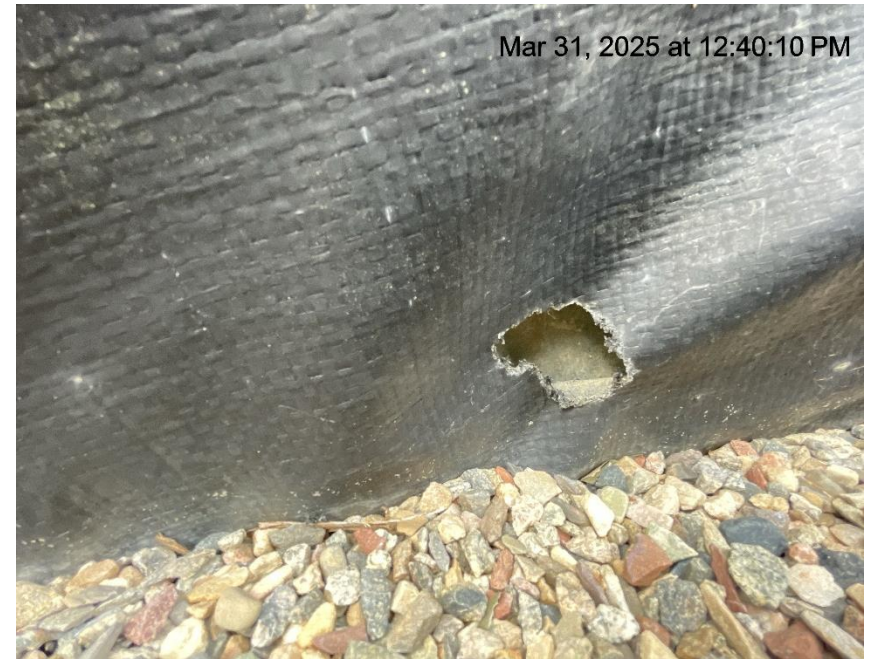
Photo # 8405 Hole in secondary containment liner/liner needs maintenance
