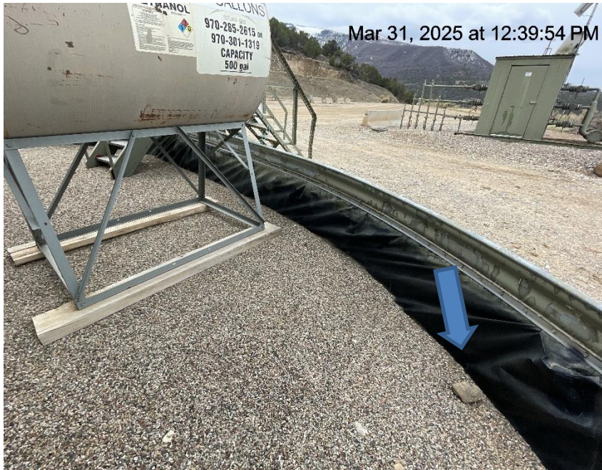
Photo # 8404 Hole in secondary containment liner/liner needs maintenance
