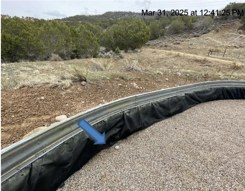
Photo # 8406 Hole in secondary containment liner/liner needs maintenance
