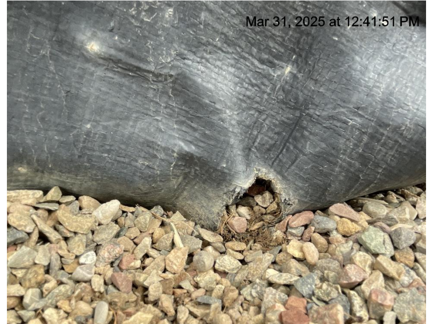
Photo # 8407 Hole in secondary containment liner/liner needs maintenance
