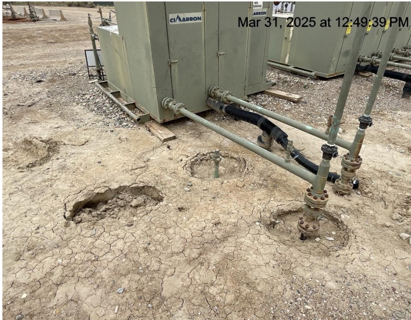
Photo # 8408 Subsidence starting to develop near separator
