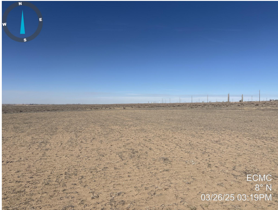
Photo 1. Photo taken from the well location, facing North. Photo illustrates that the Operator has performed final reclamation activities with evidence of drill row seeding, however vegetation establishment does not meet Rule 1004 final reclamation standards.
