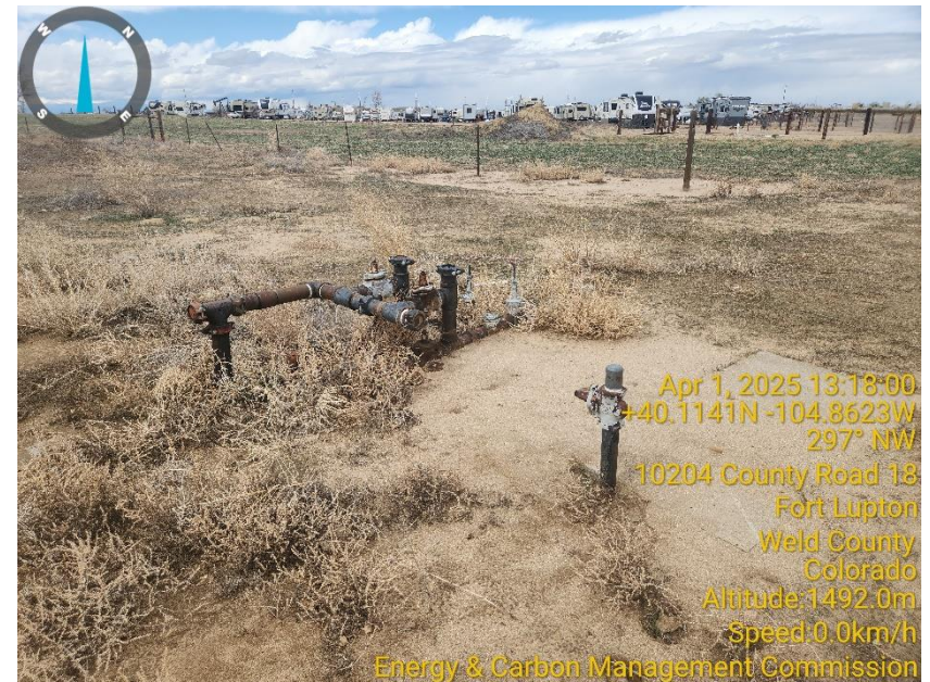
Photo 10 Flow line manifold.
