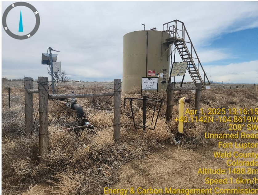
Photo 5 Gas Meter Run & tank battery.
