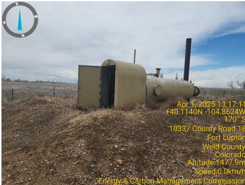
Photo 11 Horizontal Heated Separator.
