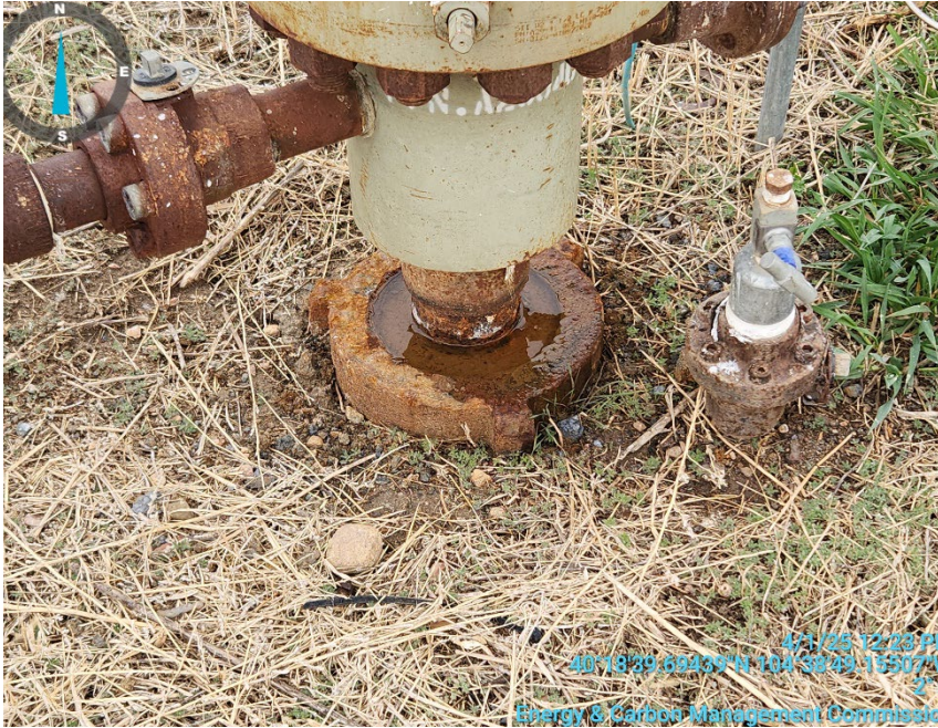
Photo 3: stained soil removed
