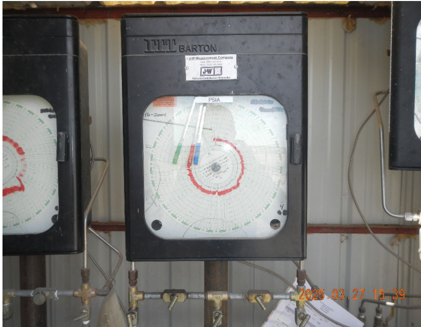
5. Gas meter inside meter shed.
