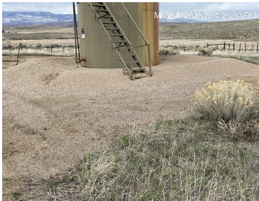
No tank battery sign. Inadequate tank containment.
