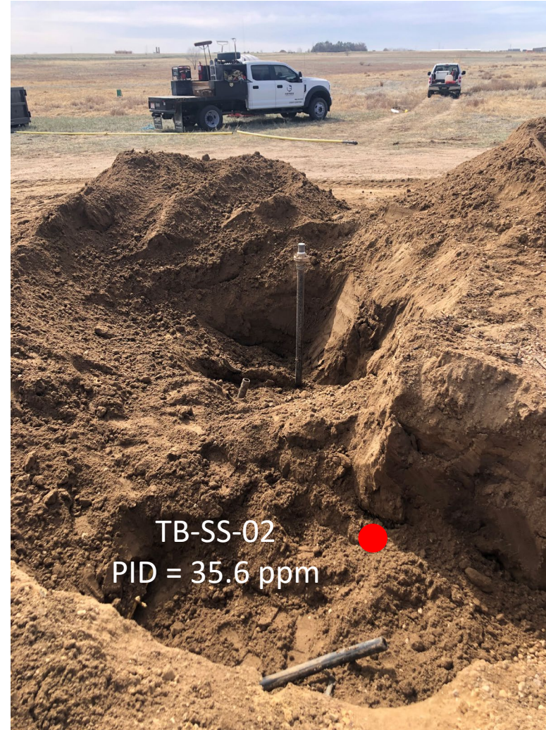
Looking south at separator dumphine
