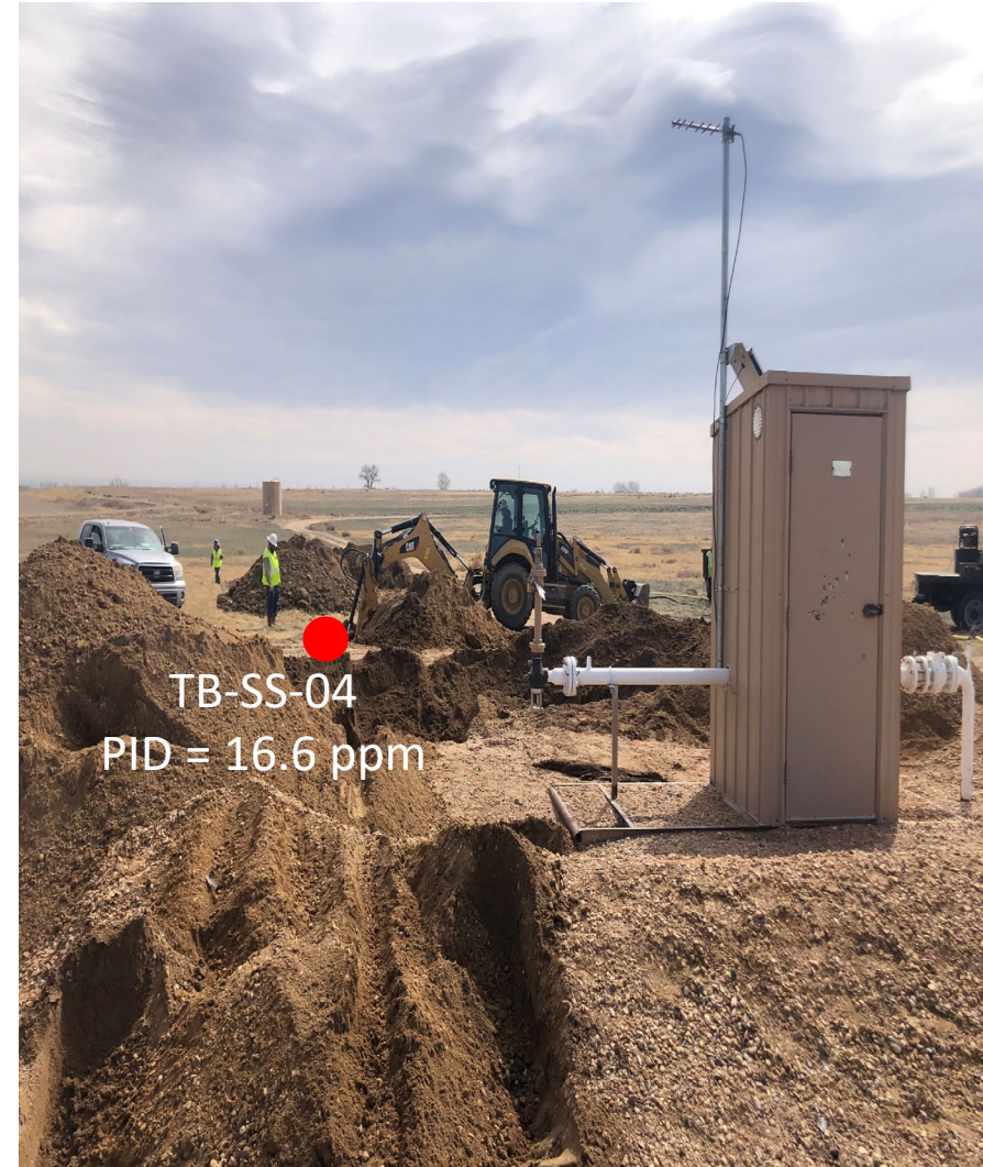
Looking east at former facility pad
