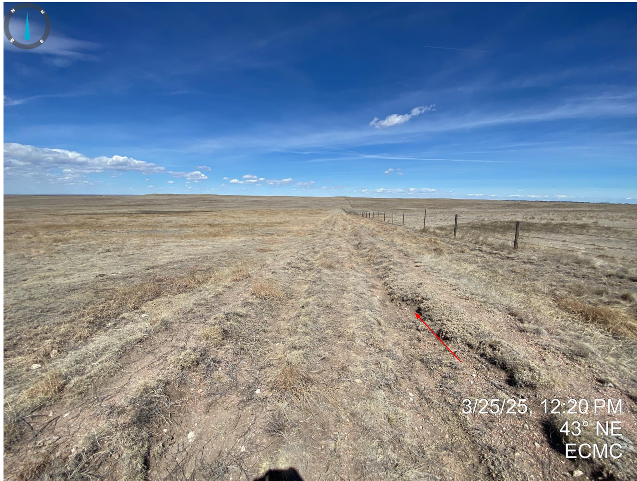
Photo 7. Taken from the northern portion of the access road. It does not appear that the access road has been reclaimed with contour/grading issues and erosion degradation evident.
