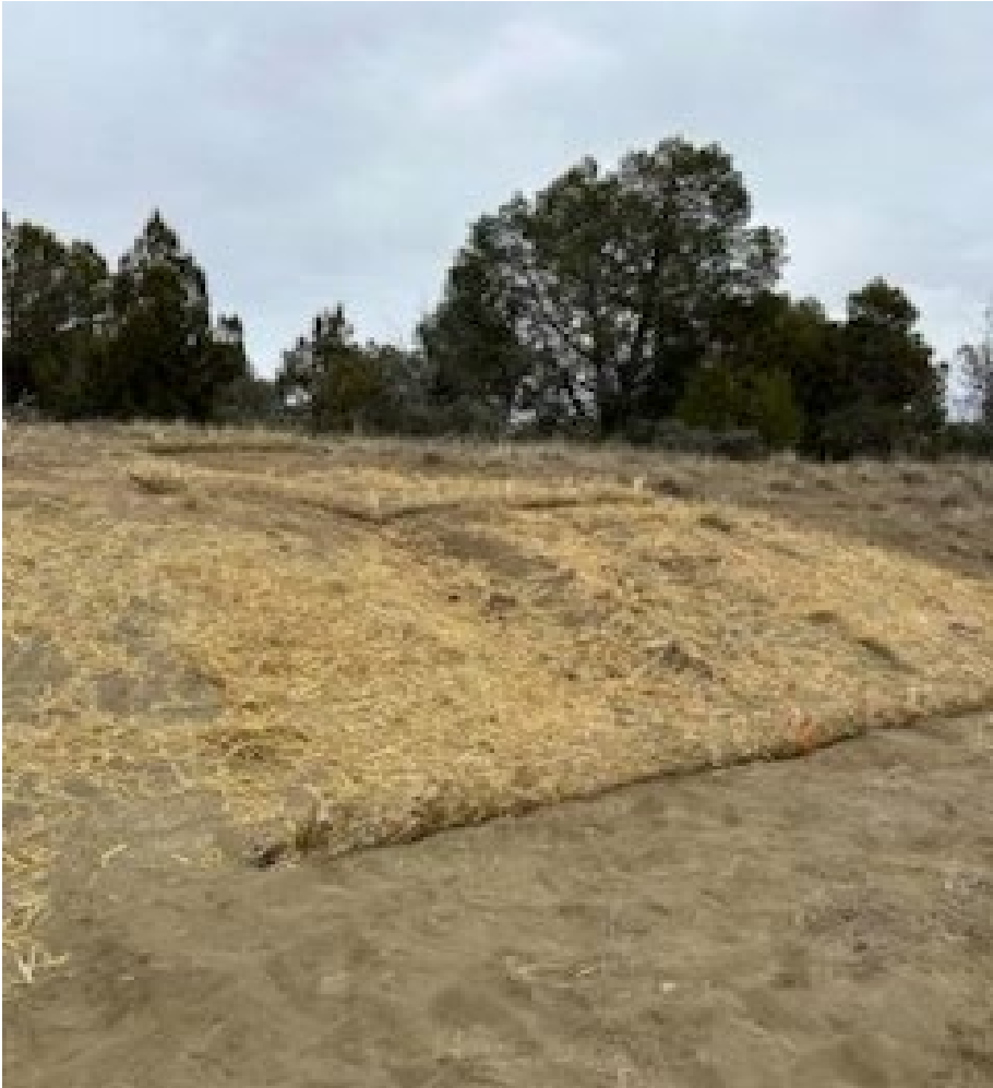
Seeding on cut slopes
