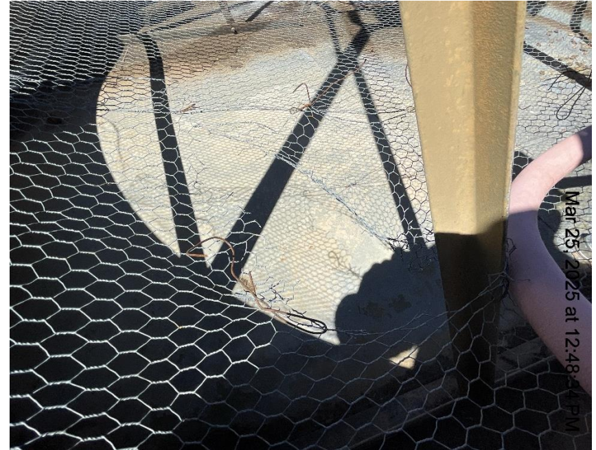
Photo # 7136 Wildlife protection on chemical tank containment needs maintenance/wildlife hazard
