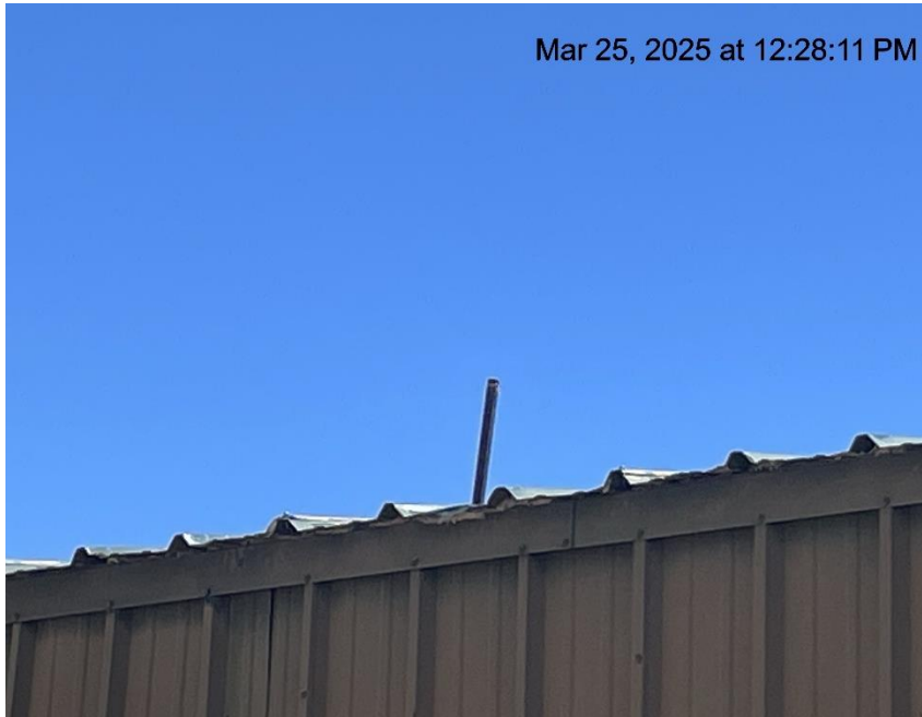
Photo # 7127 PRV vent line on compressor does not comply with CECMC pressure safety device rules
