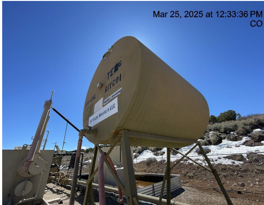
Photo # 7141 Chemical tank lacks required labeling (Additionally operator Phone # disconnected & not in service)
