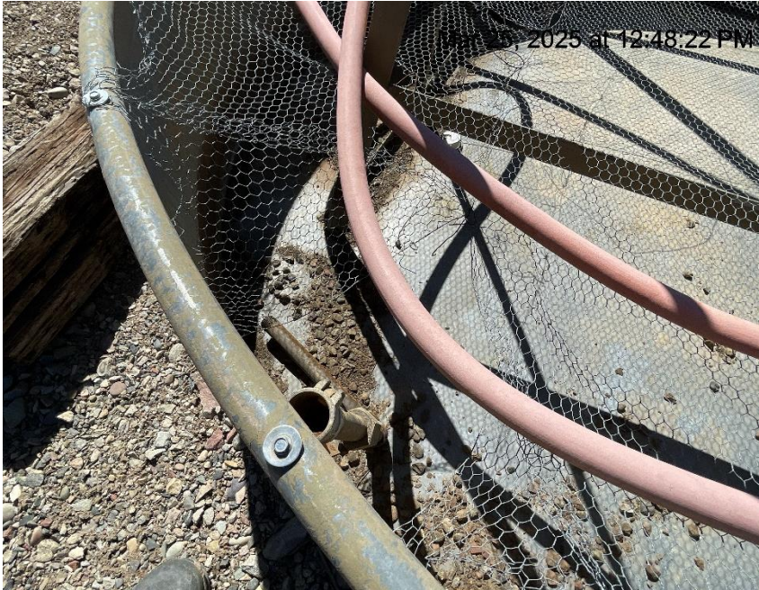
Photo # 7135 Wildlife protection on chemical tank containment needs maintenance/wildlife hazard
