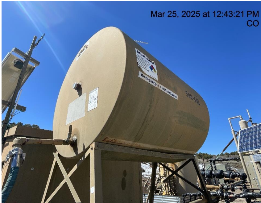
Photo # 7137 Chemical tank lacks required labeling (Additionally operator Phone # disconnected & not in service)
