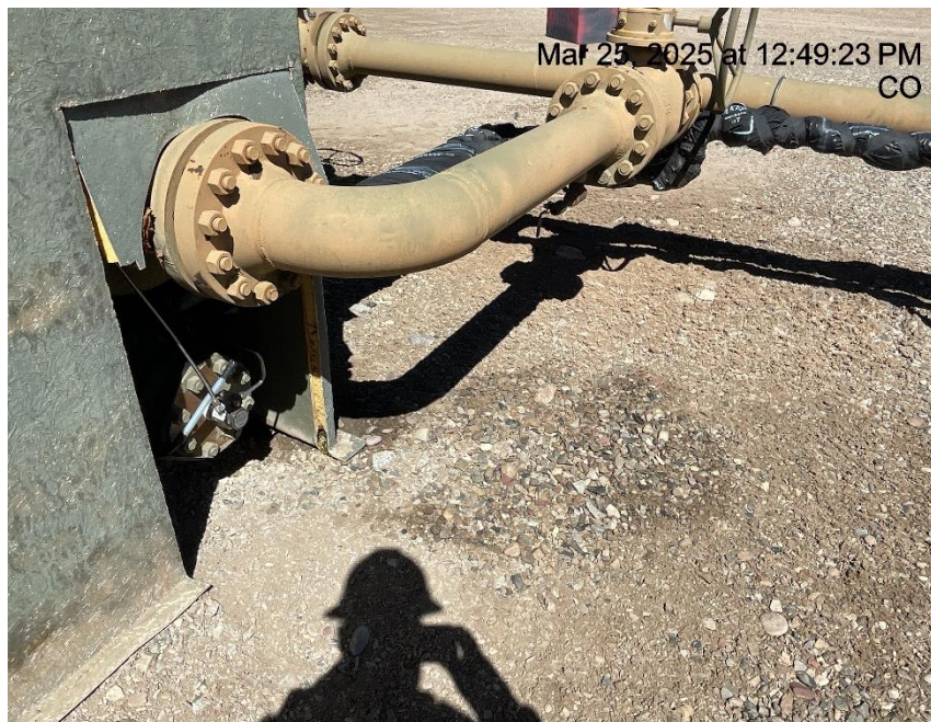
Photo # 7119 Staining near discharge coalescer
