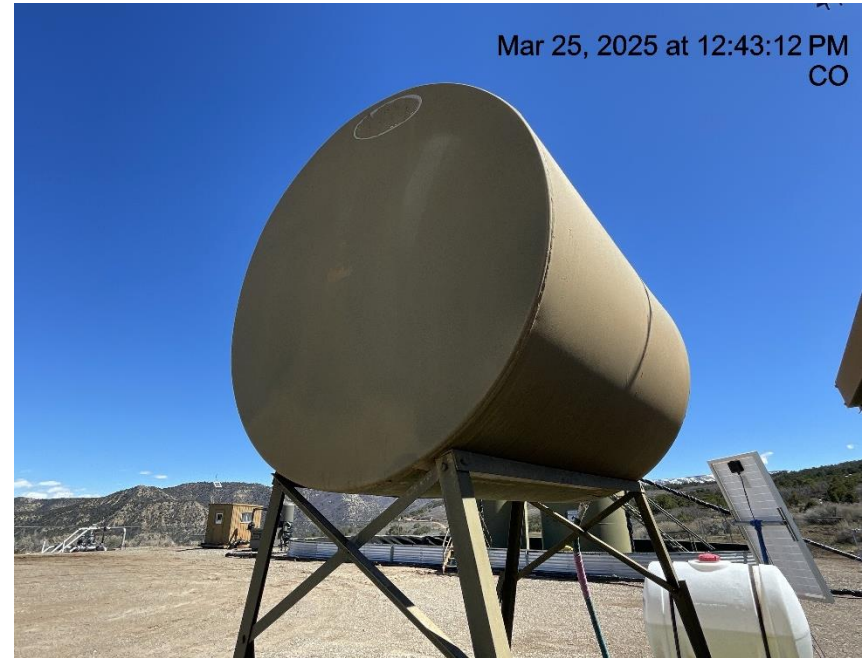
Photo # 7138 Chemical tank lacks required labeling
