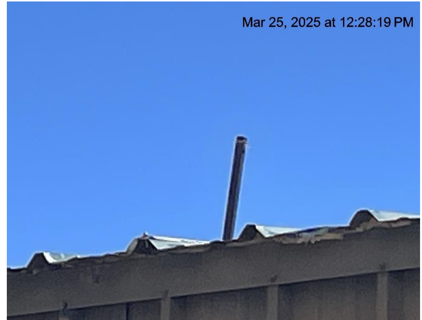
Photo # 7128 PRV vent line on compressor does not comply with CECMC pressure safety device rules
