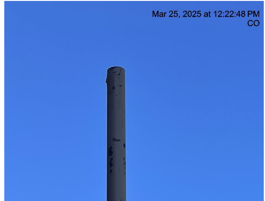
Photo # 7126 PRV vent line does not comply with CECMC pressure safety device rules
