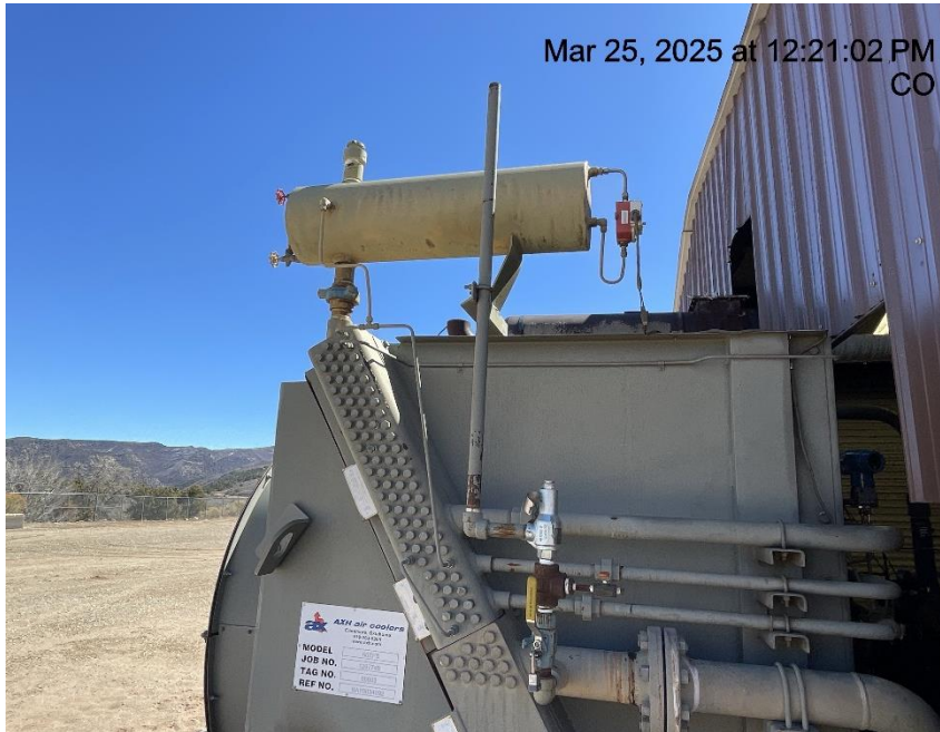
Photo # 7123 PRV vent line does not comply with CECMC pressure safety device rules
