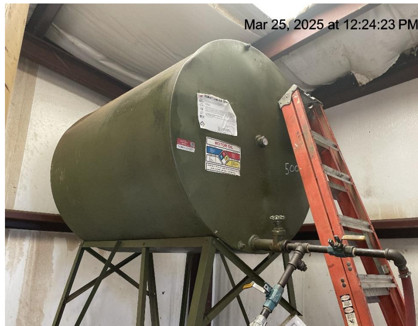
Photo # 7146 Chemical tank lacks required labeling
