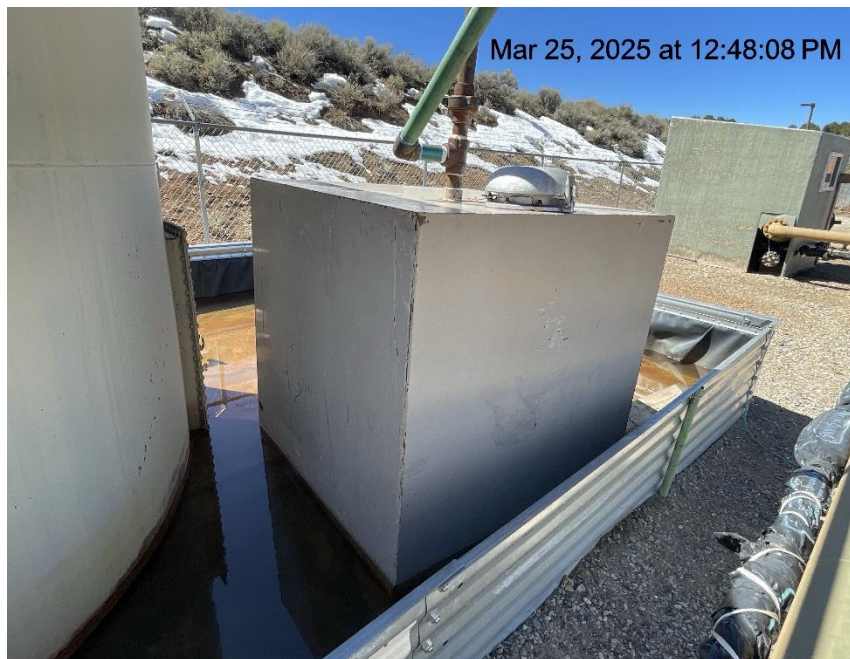
Photo # 7143 Tank lacks required labeling
