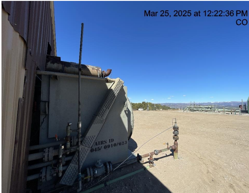
Photo # 7125 PRV vent line does not comply with CECMC pressure safety device rules
