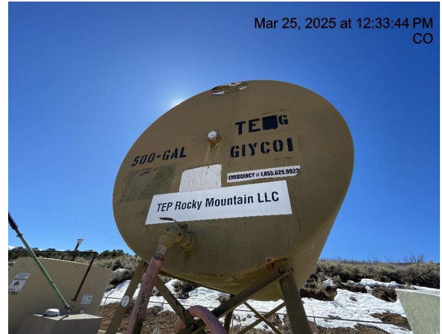
Photo # 7140 Chemical tank lacks required labeling (Additionally operator Phone # disconnected & not in service)
