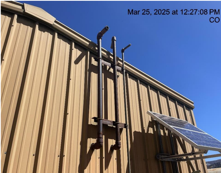
Photo # 7129 PRV vent lines do not comply with CECMC pressure safety device rules
