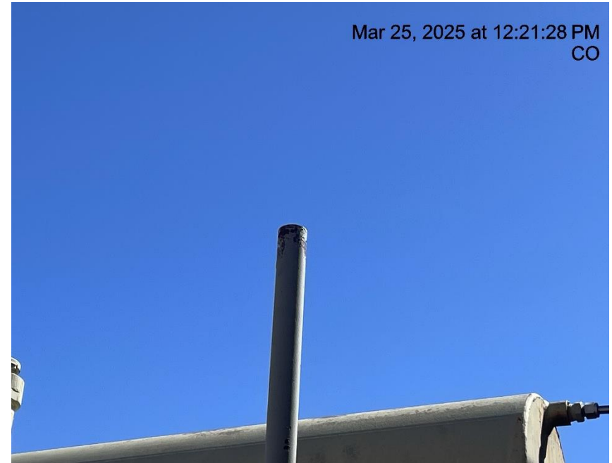
Photo # 7124 PRV vent line does not comply with CECMC pressure safety device rules
