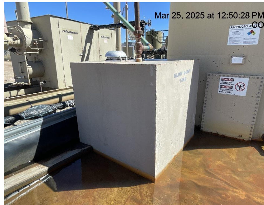
Photo # 7144 Tank lacks required labeling
