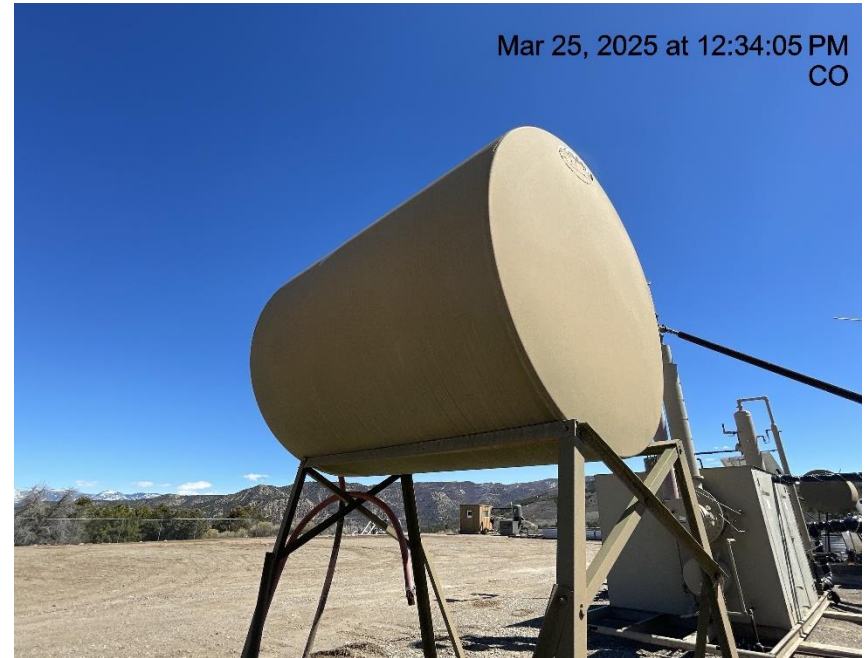
Photo # 7142 Chemical tank lacks required labeling
