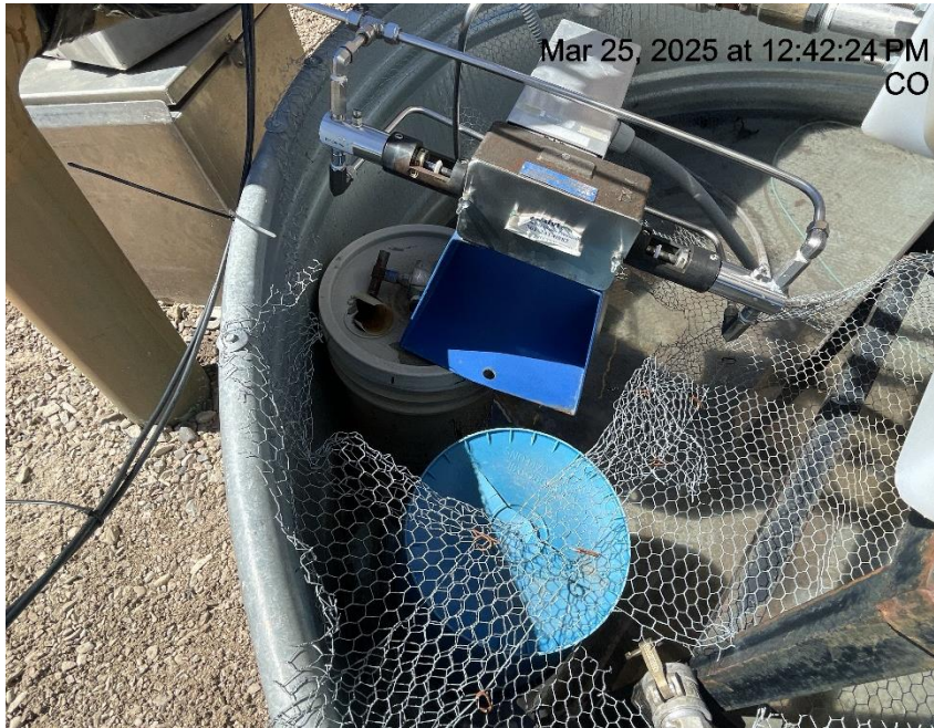
Photo # 7133 Wildlife protection on chemical tank containment needs maintenance/wildlife hazard
