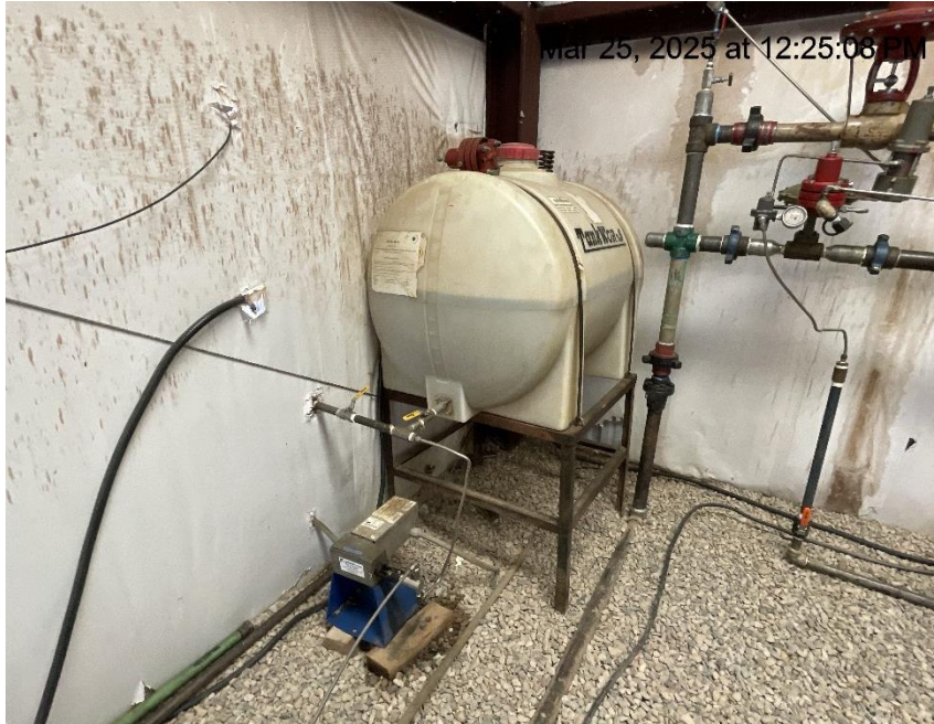
Photo # 7148 Chemical tank in compressor building lacks BMP's
