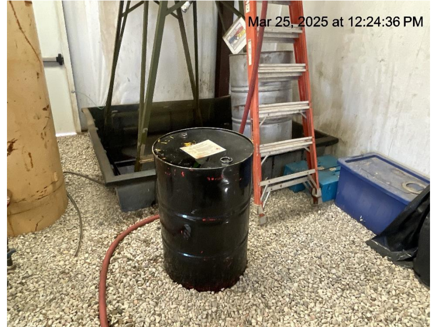
Photo # 7149 Chemical drum in compressor building lacks BMP's
