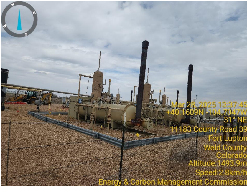
Photo 3 Horizontal Heated Separators.
