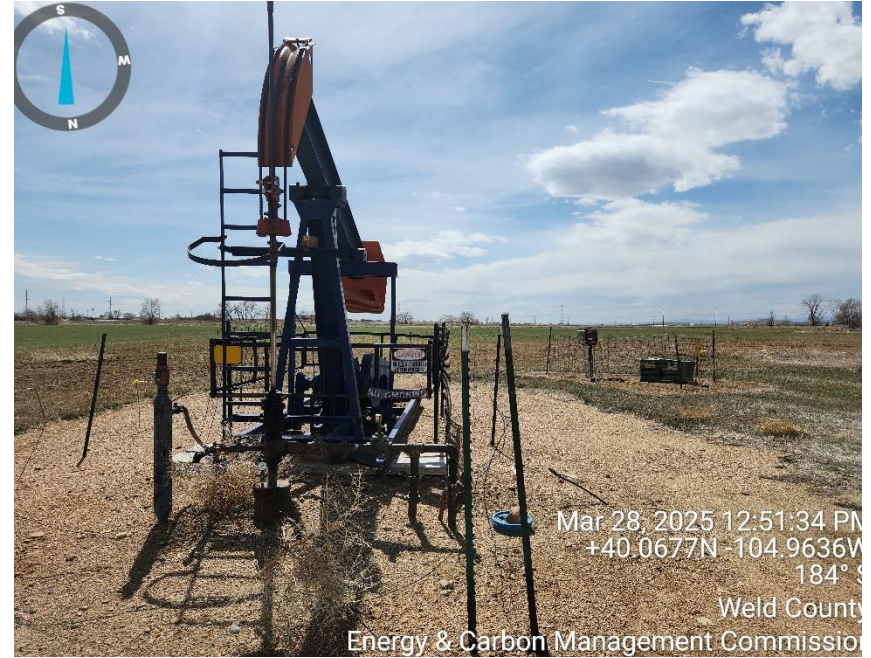
Photo 2 well head and equipment
