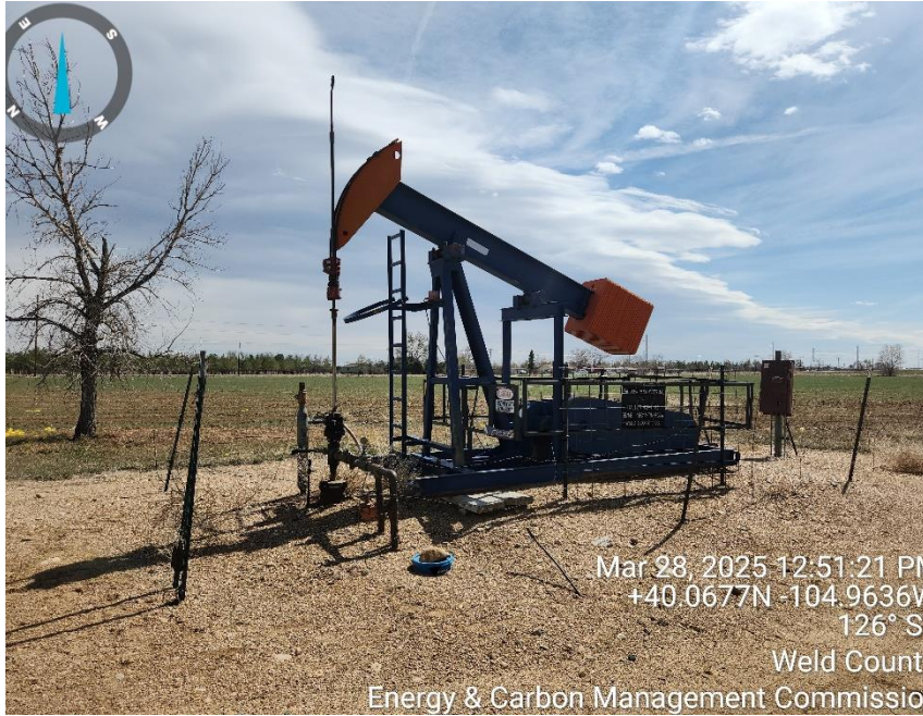
Photo 1 well head and equipment
