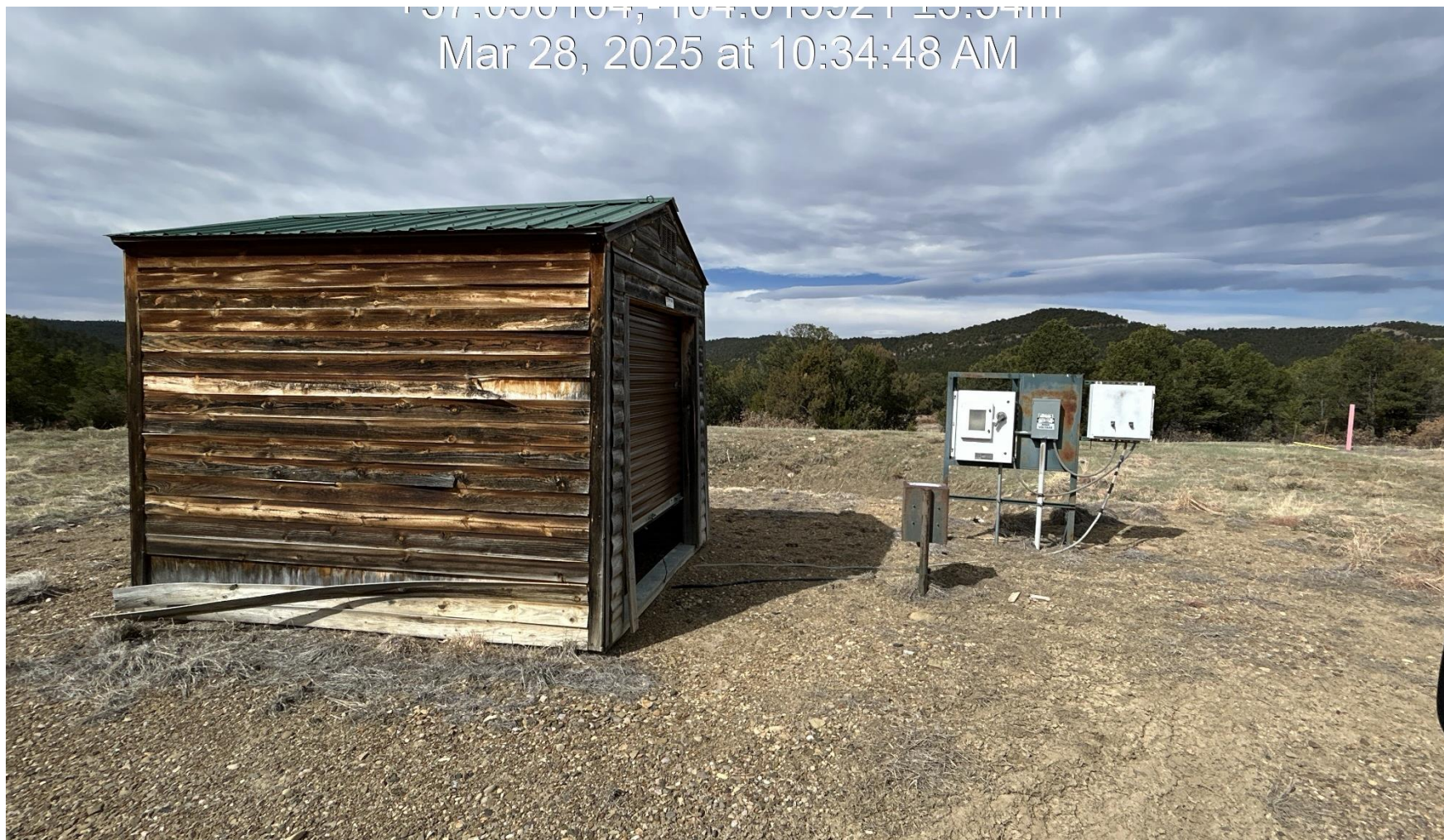
PHOTO 3: WELLHEAD AND EQUIPMENT
