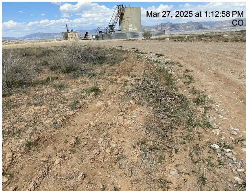
Photo # 8027 Failure to minimize surface disturbance
