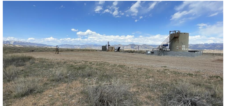
South East corner of location.
