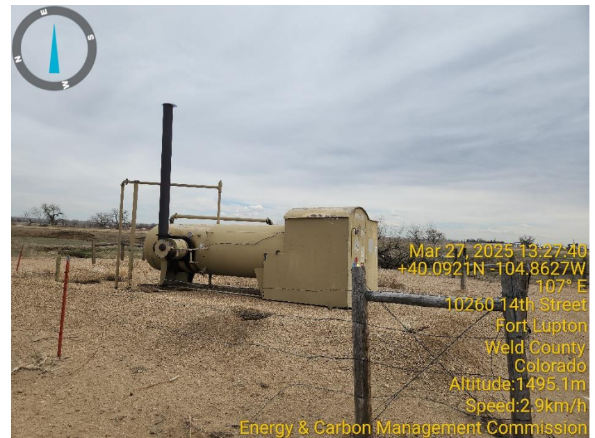
Photo 2 Horizontal Heated Separator.
