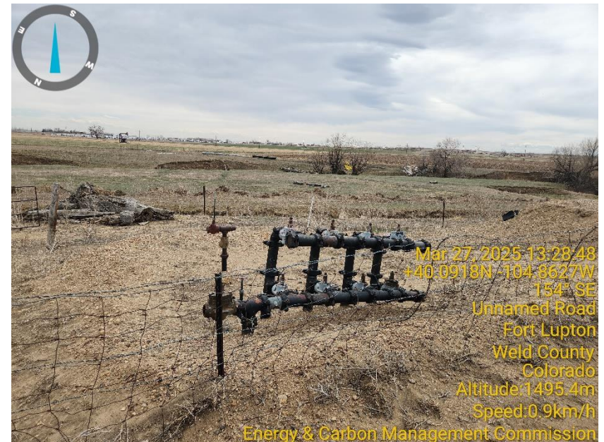
Photo 4 Flow line manifold.
