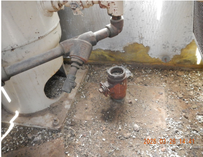
5. Open ended lines inside meter shed.
