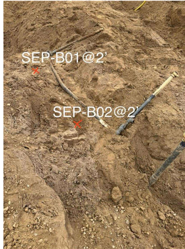
Separator soil samples facing north.
