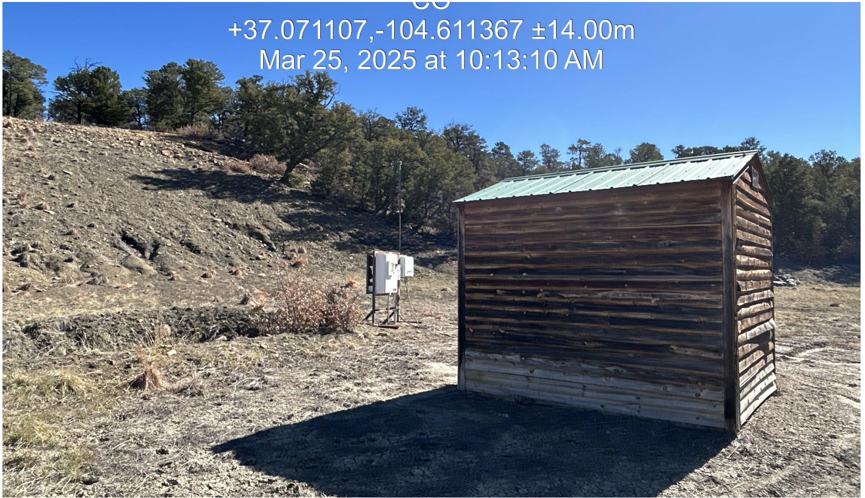
PHOTO 3: WELLHEAD AND EQUIPMENT
