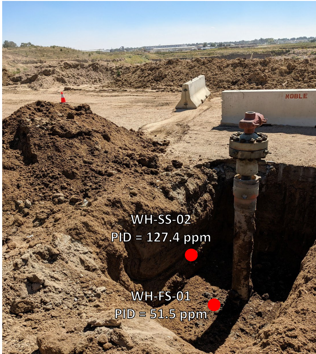
Looking southeast No petroleum hydrocarbon staining or odor observed
