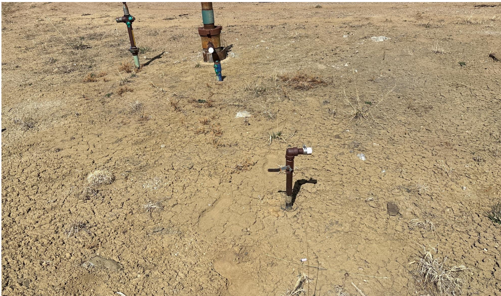
PHOTO 4: 1' RISER IS NOT MARKED. ALL UNUSED RISERS MUST BE CLEARLY MARKED OR REMOVED PER RULE 606. THIS IS THE SECOND NOTICE FOR THIS RISER IMMEDIATE ACTION IS REQUIRED.
