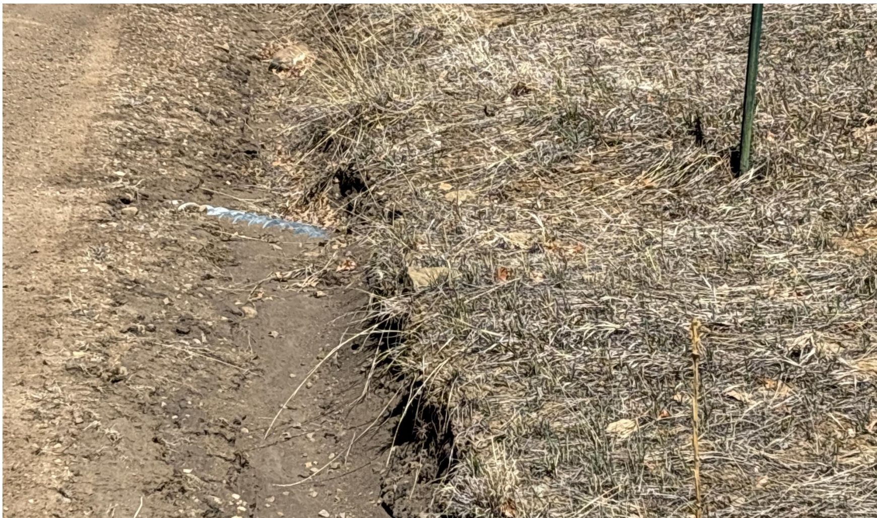
PHOTO 4: CULVERT NORTHWEST OF LOCATION IS SILTED IN ON BOTH ENDS. CLEAN AND MAINTAIN EMP'S PER RULE 1002. CA DATE 4/8/2025.
