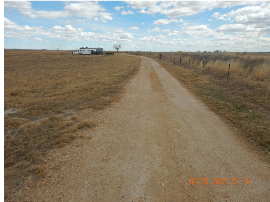
Photo 5. Photo taken from a portion of the western access road, facing West. Photo illustrates the access road has been left graveled and stabilized. At the time of this inspection, there were no stormwater erosion issues.
