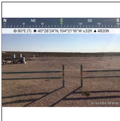
P2 - Looking east from the center of the Site excavation. The facility has returned to production following the excavation.
