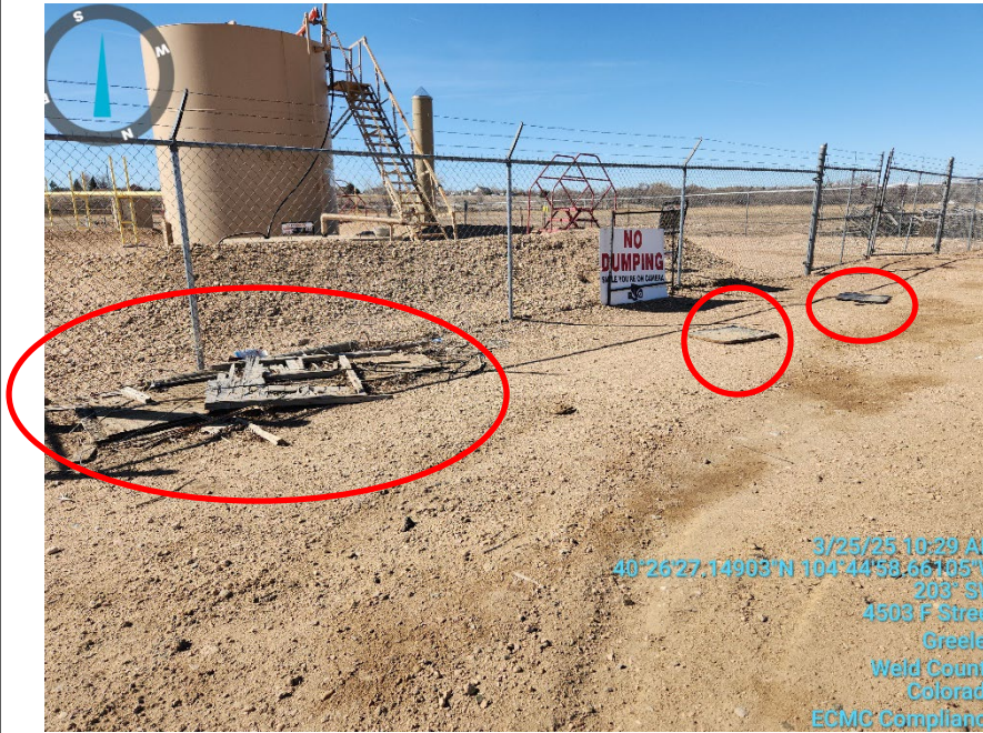
Photo 9: Trash and debris
