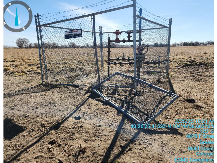
Photo 4: Fencing in disrepair
