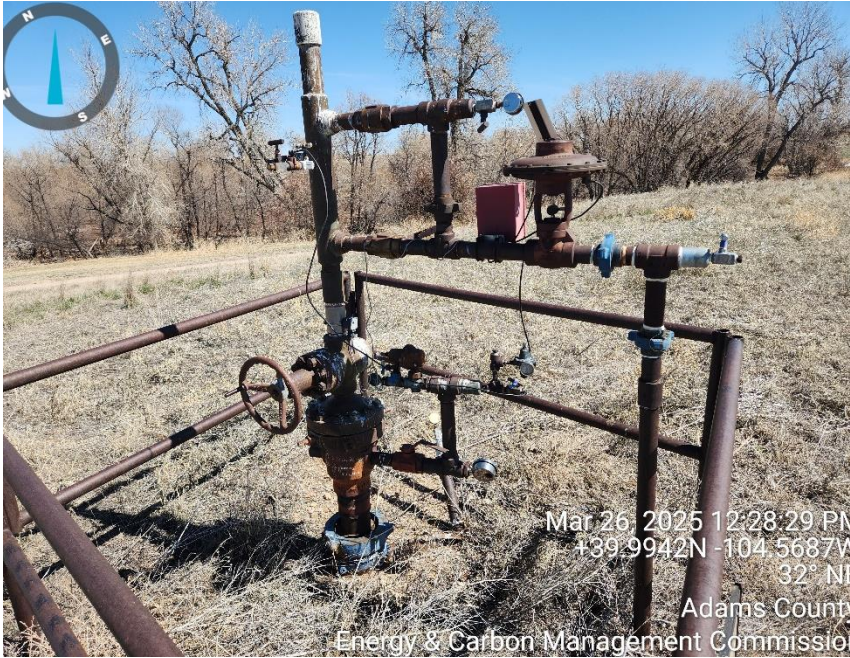
Photo 2 well head and equipment
