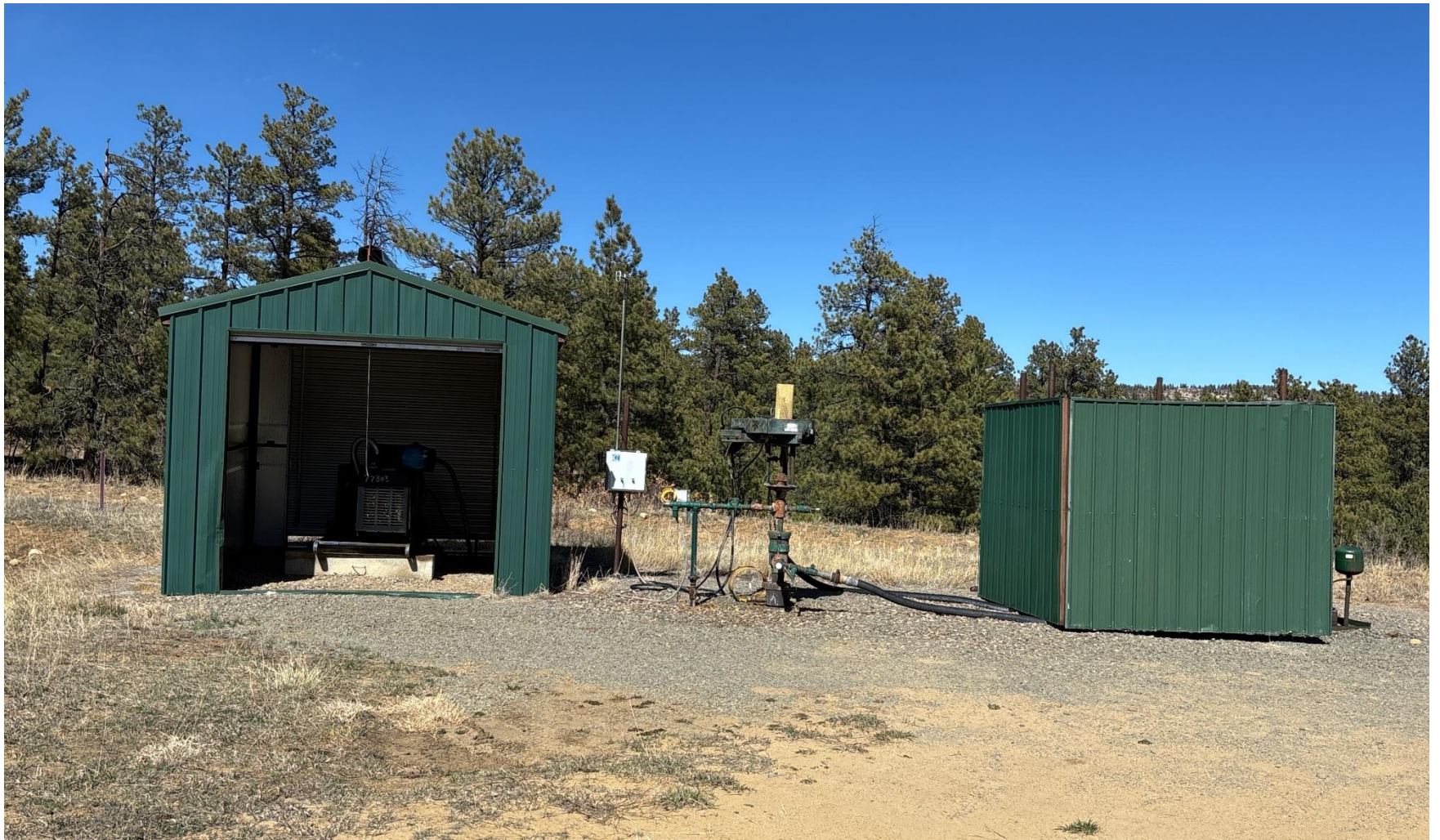
PHOTO 3: WELLHEAD AND EQUIPMENT.
