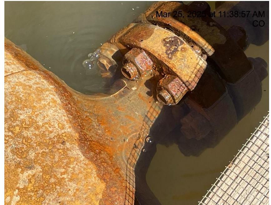
Photo # 6886 Mechanical Condition - Possible leak on CSF 44C-09-07-91 wellhead
