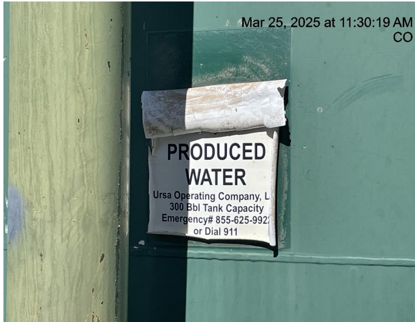
Photo # 6897 Tank label contains inaccurate information
