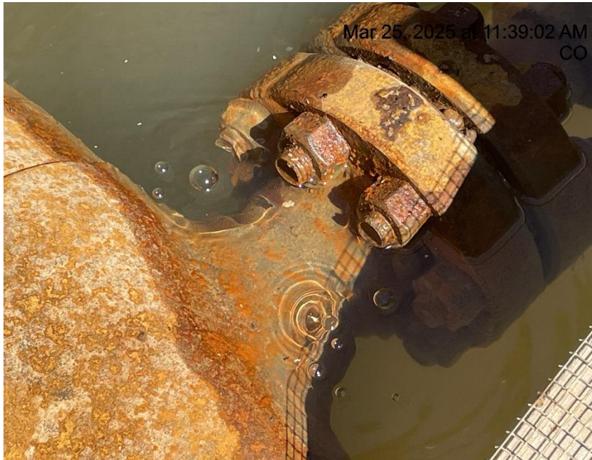
Photo # 6885 Mechanical Condition - Possible leak on CSF 44C-09-07-91 wellhead
