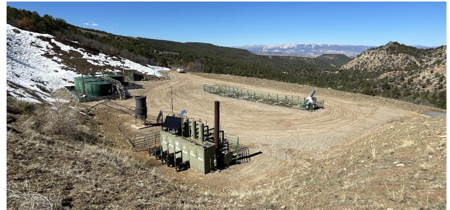
South East corner of location.
