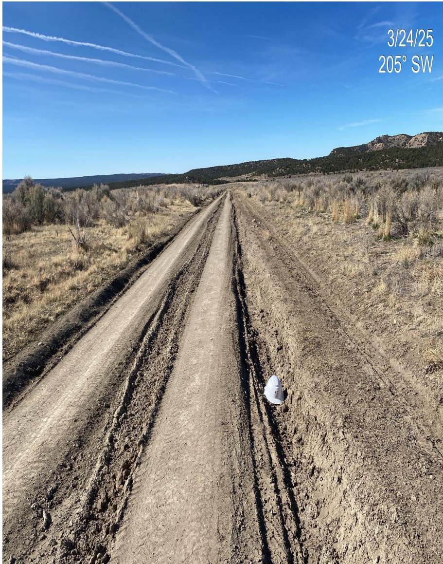
Photo 6. Rutting (ranging 10-14 inches in depth) observed along length of access road approaching well pad.
