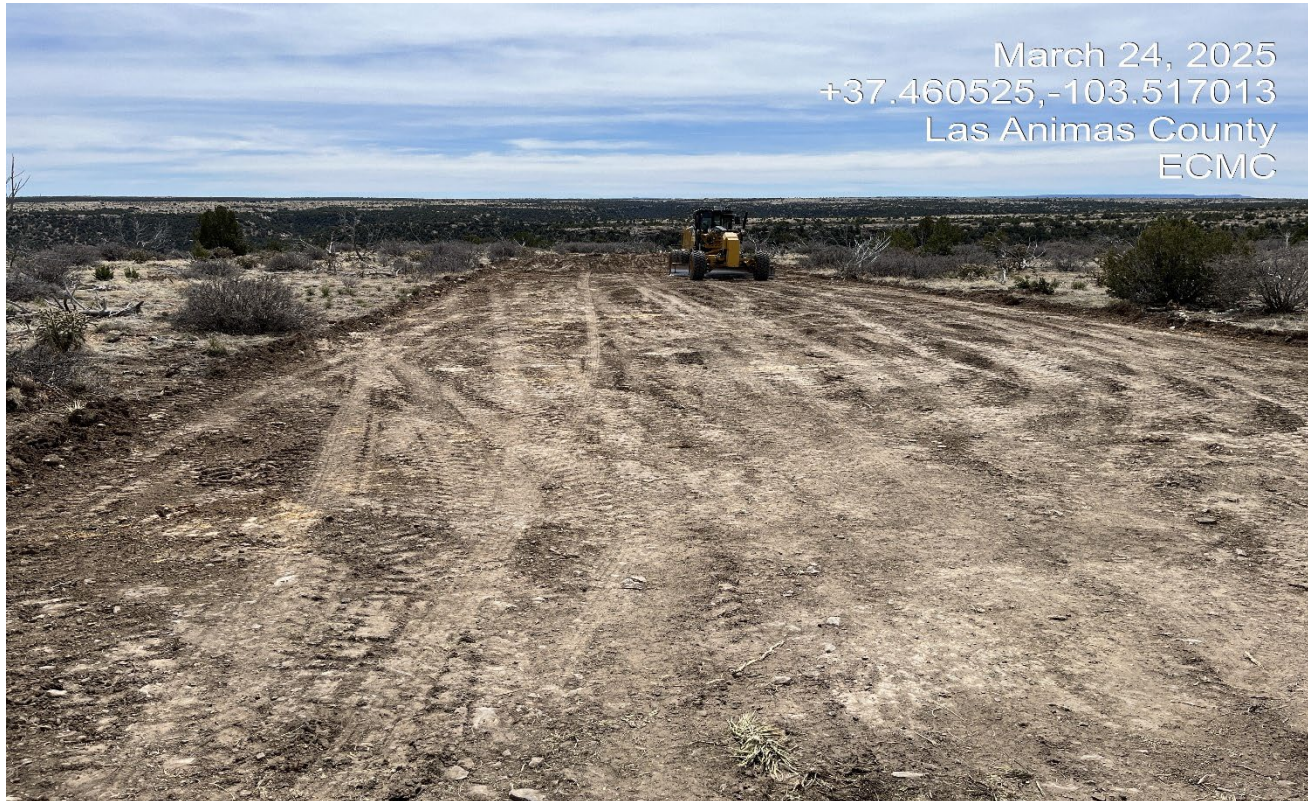
Photo 4. Facing south at the location. Topsoil has been salvaged from the location.
