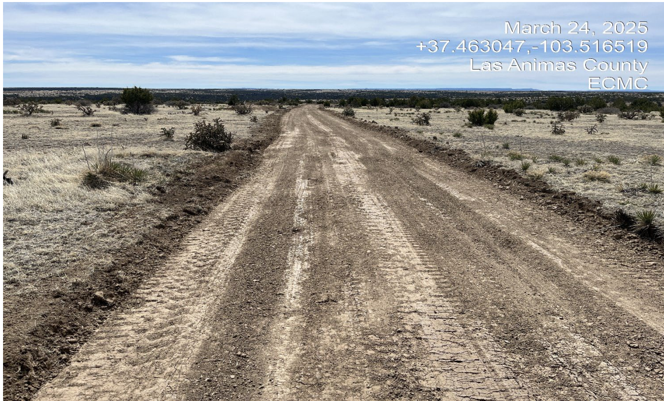
Photo 1. Facing south along the access road. Topsoil was salvaged along the road.
