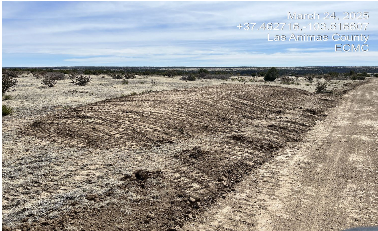
Photo 2. Facing toward the topsoil pile salvaged along the road. The topsoil will need to be seeded for long term stabilization..
