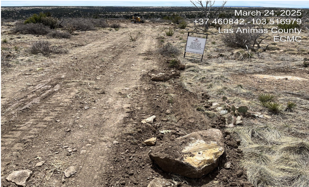
Photo 3. Facing south near the location. This portion of the road was very rocky and topsoil was not salvaged at this area.
