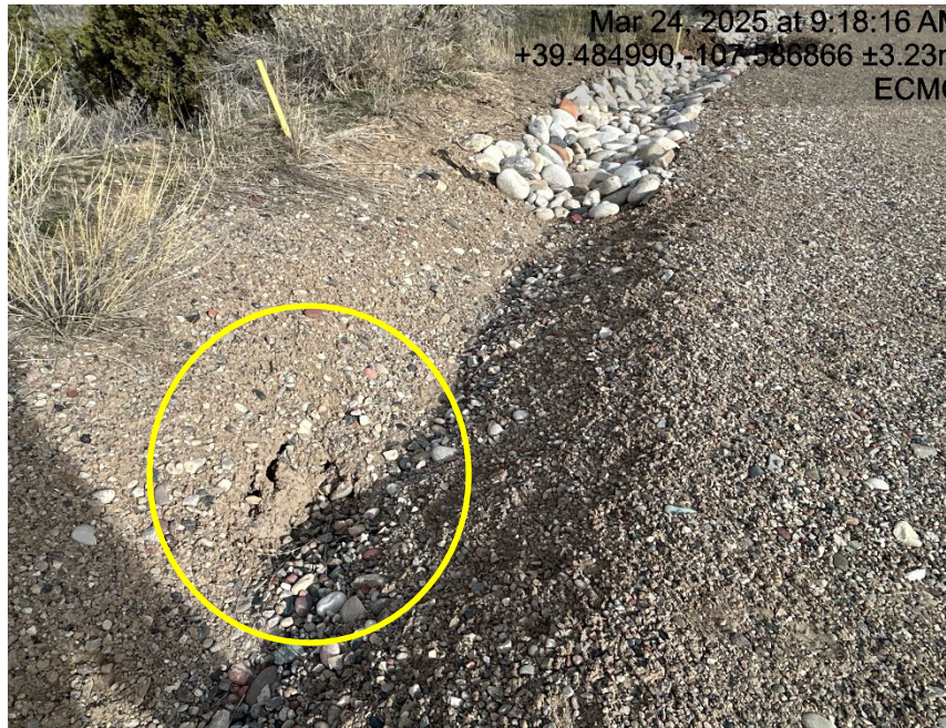
Subsidence in ditch/berm
