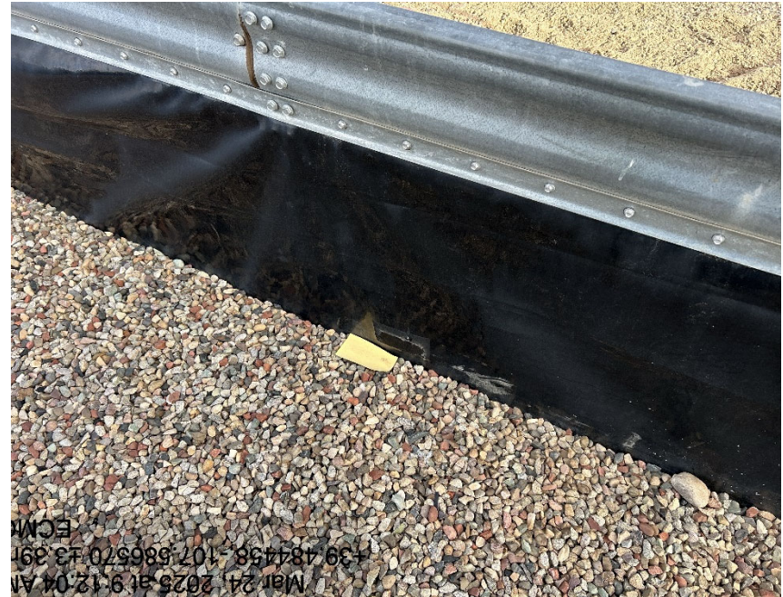
Hole in containment
