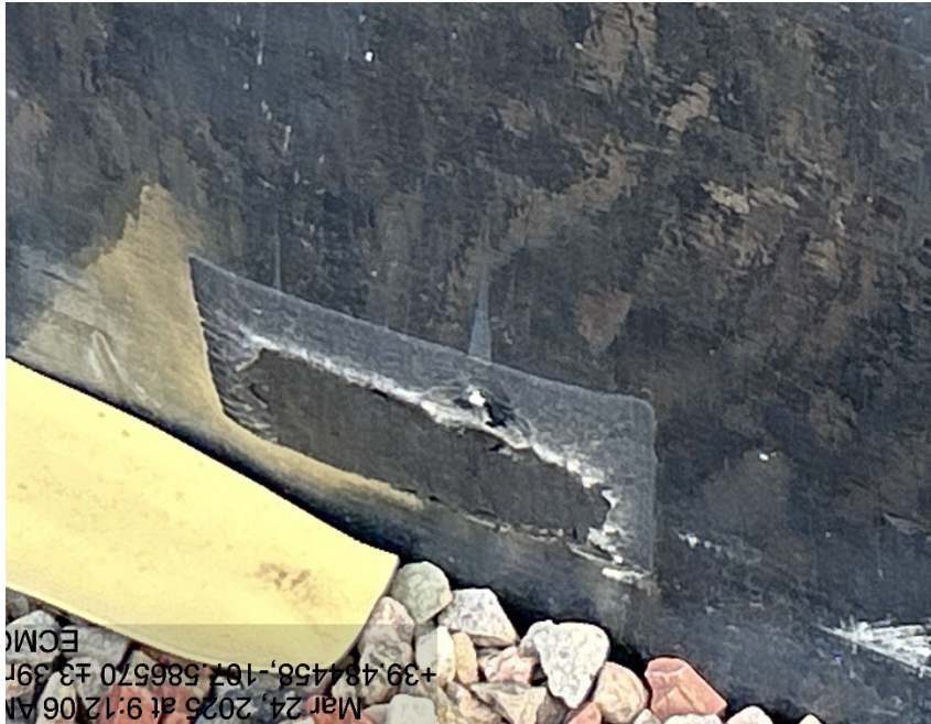
Hole in containment
