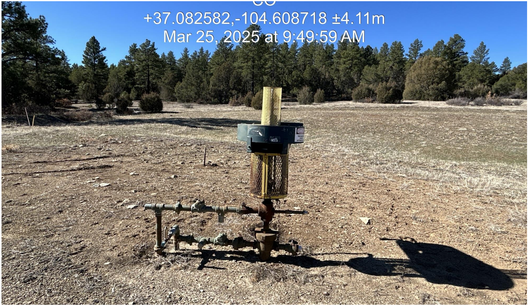
PHOTO 3: WELLHEAD AND EQUIPMENT
